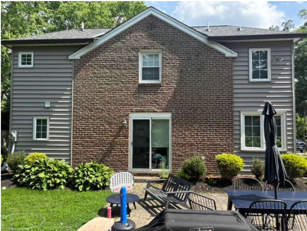
Figure 4. View of 12 Barley Cone Lane Rear, Facing South
