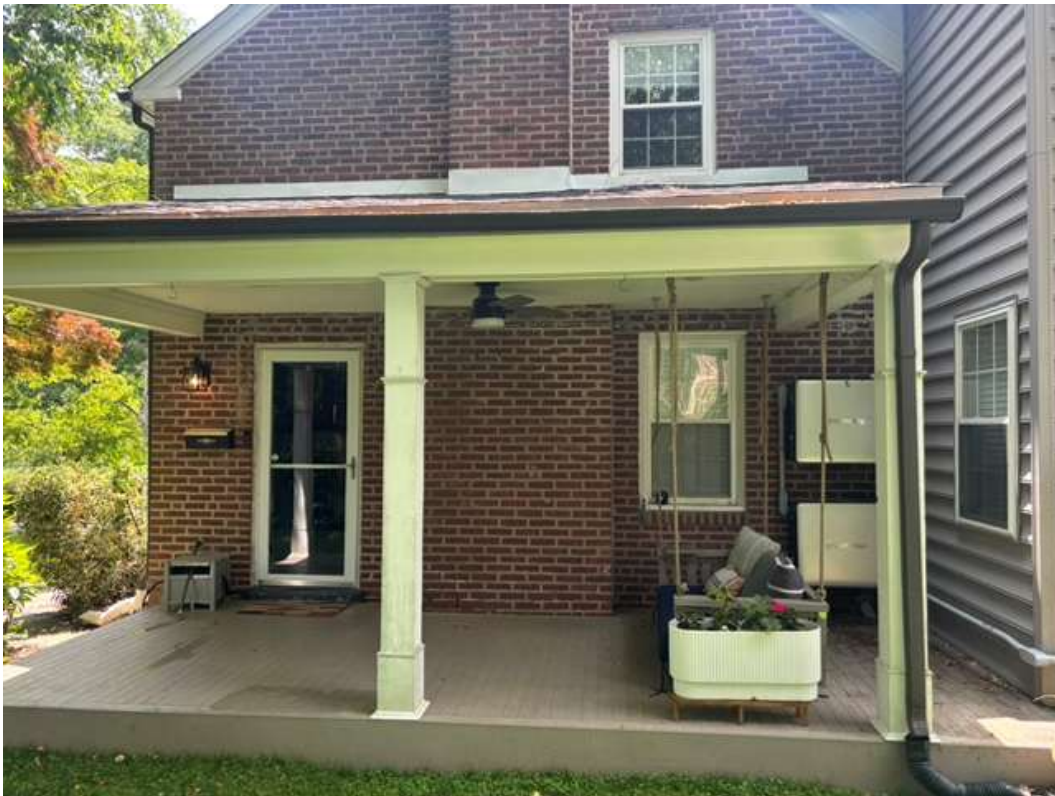
Figure 6. View of 12 Barley Cone Lane Side and Front Door, Facing West
