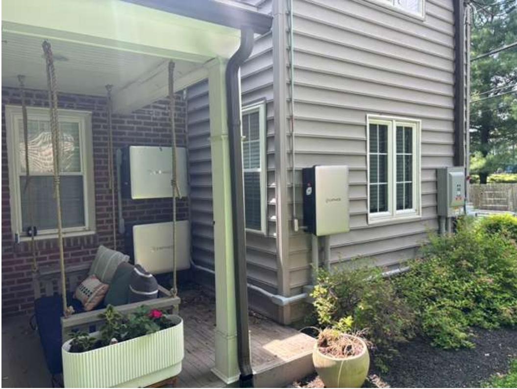
Figure 7. View of 12 Barley Cone Lane Side, Facing West
