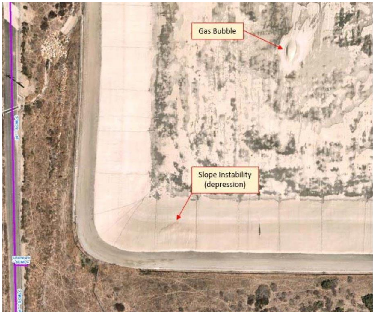
Pond 1/2 Areas of Mechanical Failure
