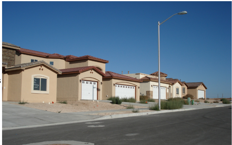
A look at the new houses being built in Camino Crossing.
