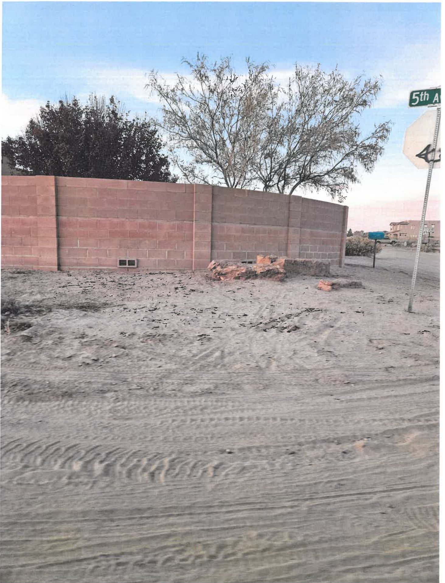
South East facing wall
