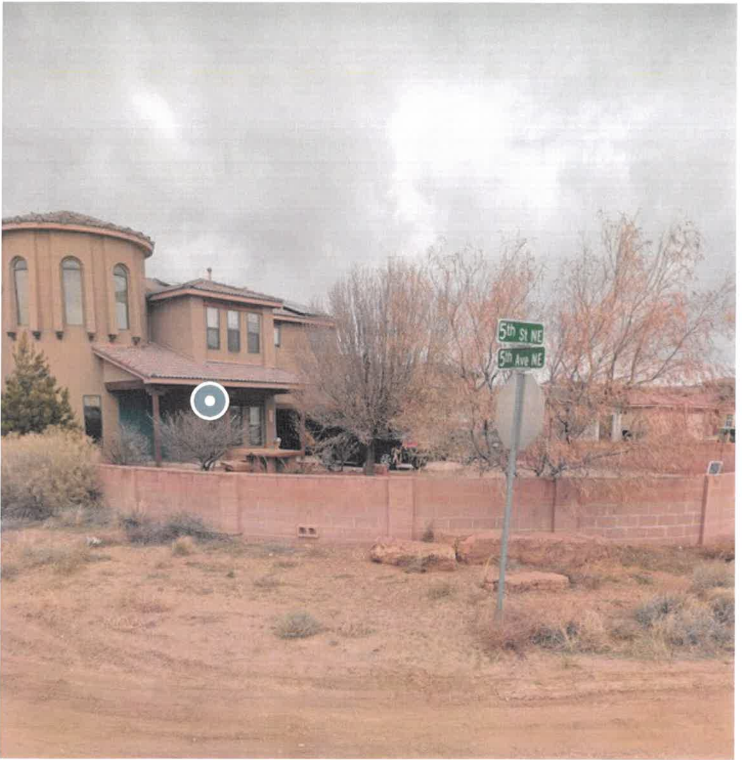
Corner of property BEFORE raising wall
