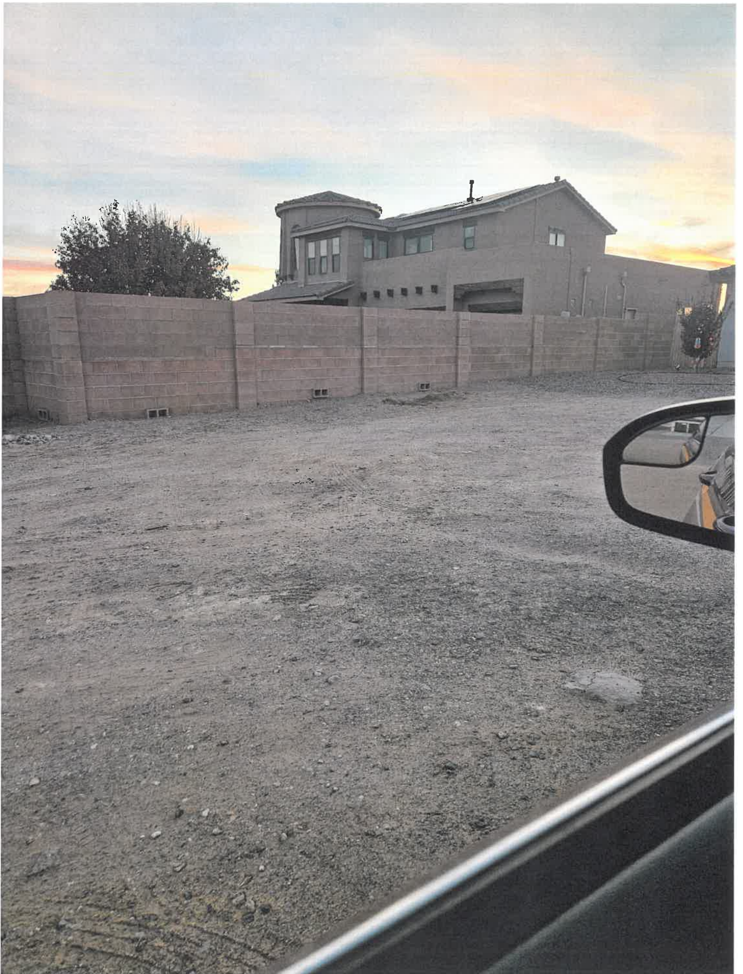
North side of wall shared with 405 5th St. Neighbors
