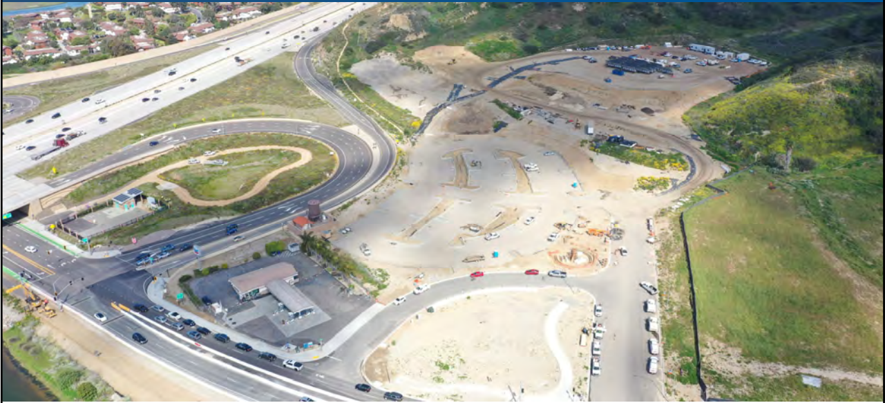
Current construction status – April 2023
