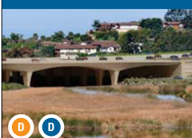
Lagoon Bridge Replacements*
