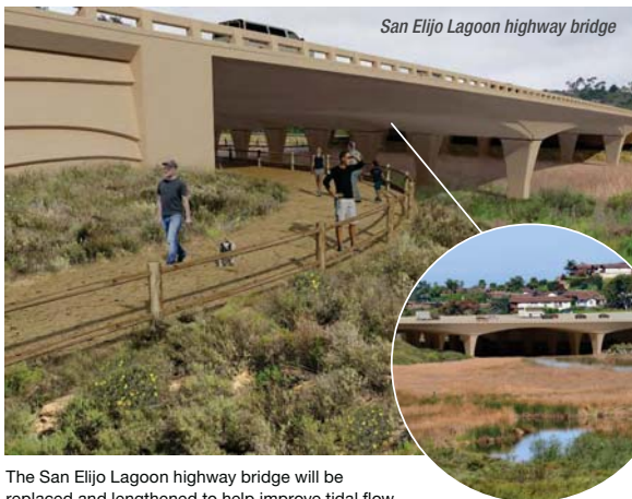
San Elijo Lagoon highway bridge
