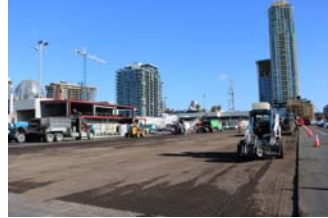
IAD Repaving Project
