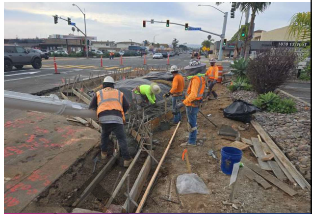
Placing concrete for trench drain system
