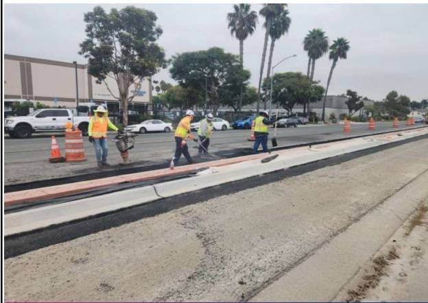
Placing asphalt concrete for slot paving on Beyer Blvd south of Dairy Mart Rd.
