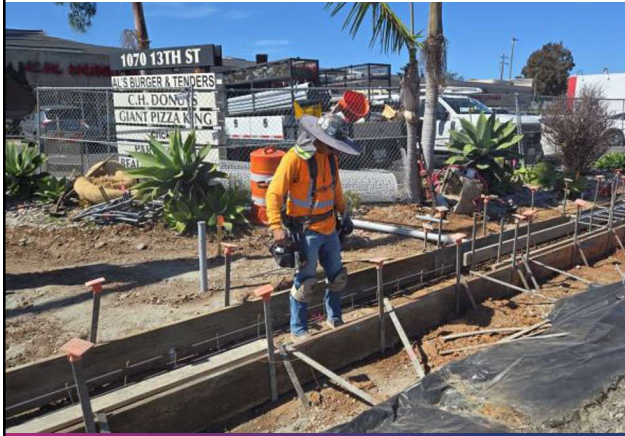
Setting rebar for trench drain system
