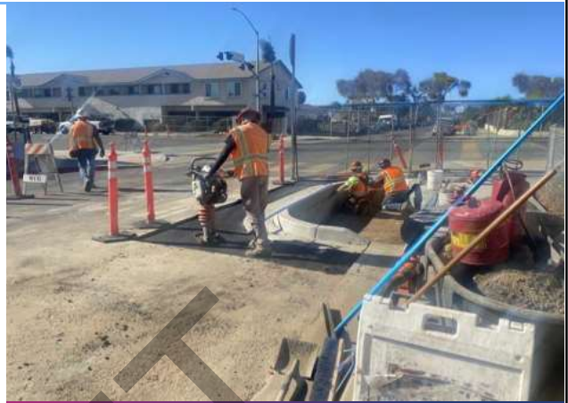
Placing asphalt concrete pavement at SW corner of 13th St and Grove Ave.
