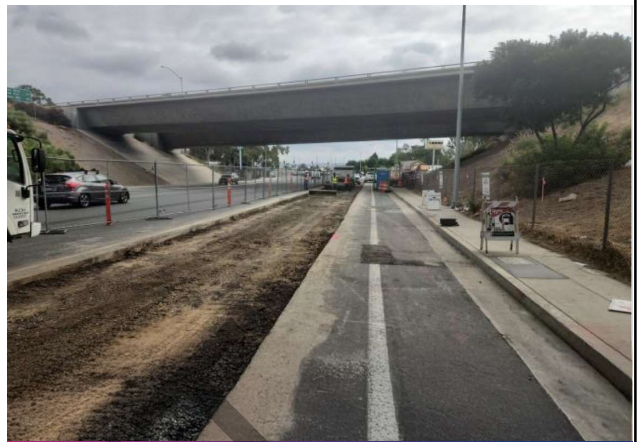
Subgrade preparation Saw-cutting existing pavement on Beyer Blvd at Iris Ave.
