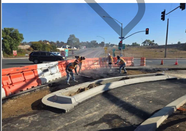
Placing AC for slot paving at Beyer Blvd and Iris Ave.
