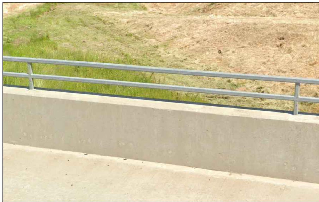
GALVANIZED STEEL HAND RAILING ABOVE THE CONCRETE SIDEWALK BARRIER
