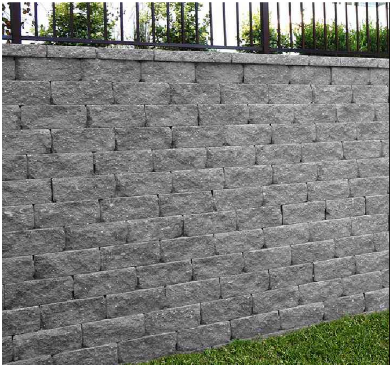
GRAY BLOCK AT APPROACH RETAINING WALLS
