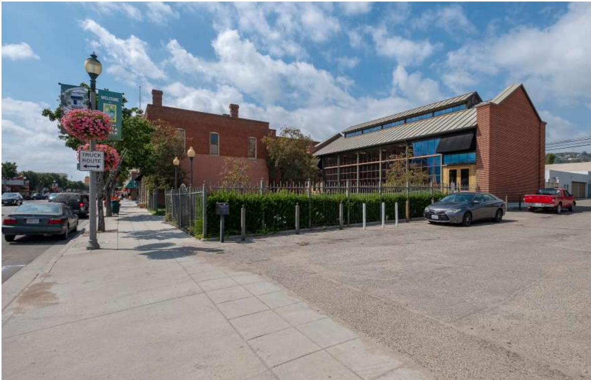
Existing Vacant Lot (Parking Area)
