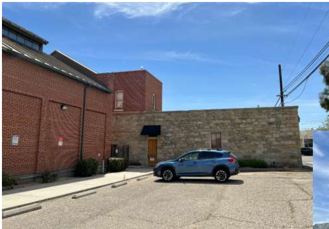
Existing Parking Area
