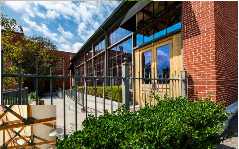
Oil Rig Building South Facade
