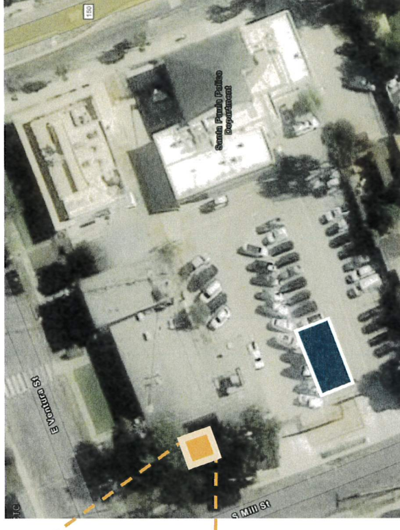
Aerial image of the solar and battery location
