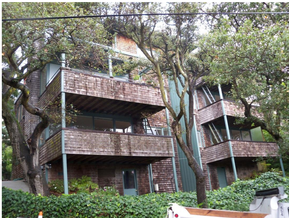
Figure 92. 30 Excelsior Lane, 2013 Source: Christopher VerPlanck
