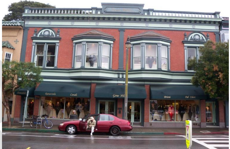
Figure 45. Former Sausalito City Hall, 731 Bridgeway. Source: Christopher VerPlanck
