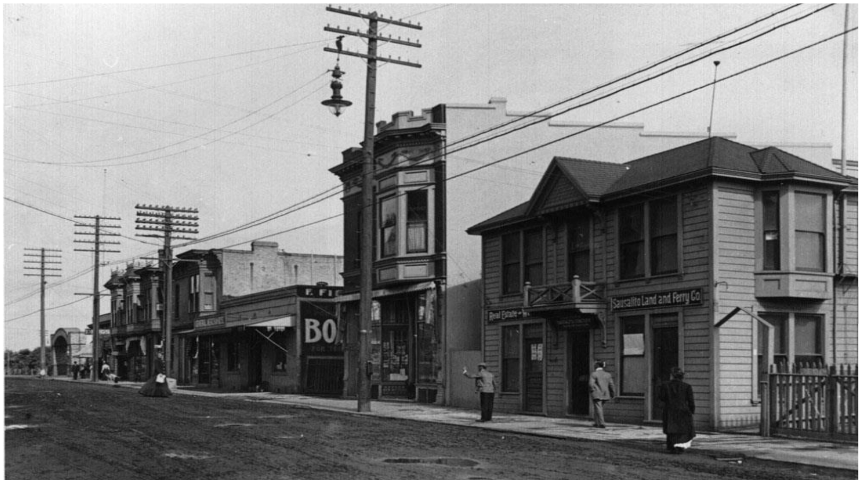
Figure 44. East side of Water Street, north of Princess Street, ca. 1910.
