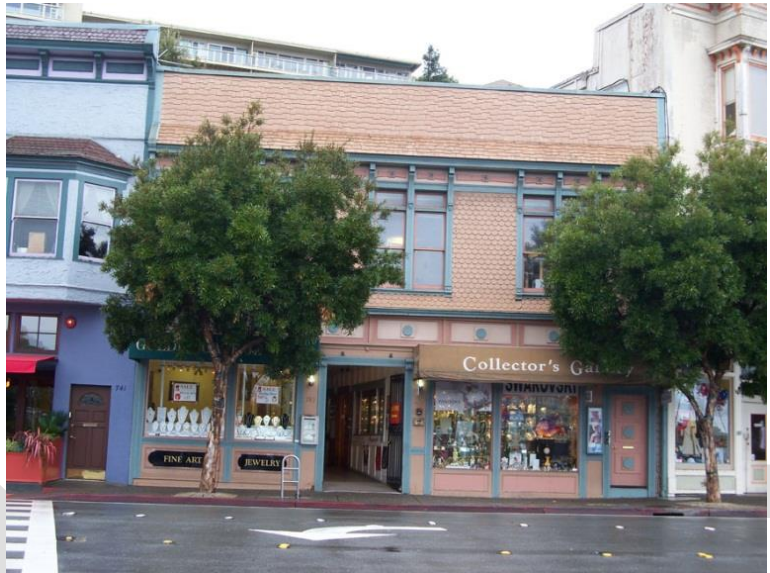
Figure 59. Arcade Shops building, 743-45 Bridgeway. Source: Christopher VerPlanck
