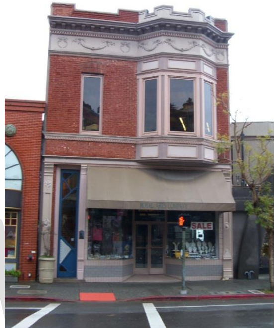
Figure 60. Becker Building 666-68 Bridgeway. Source: Christopher VerPlanck
