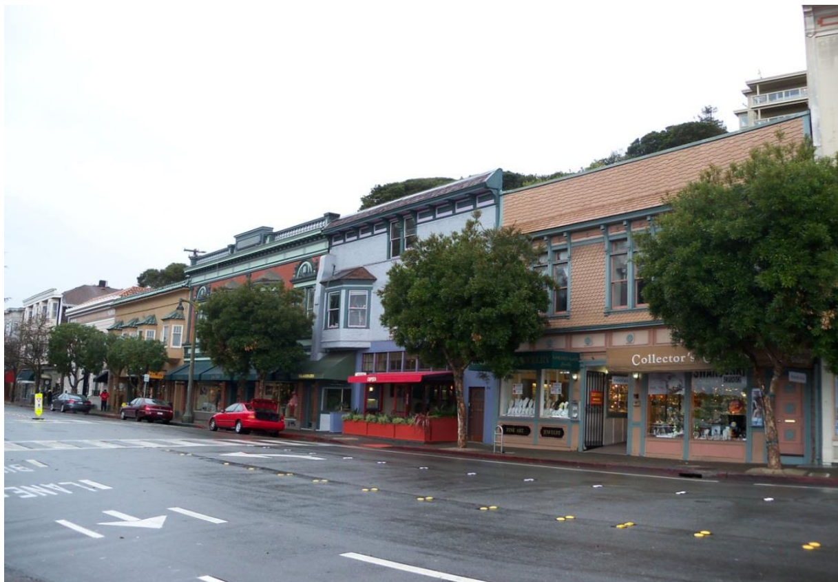
Figure 32. Commercial blocks lining the 700 block of Bridgeway, looking southwest. Source: Caitlin Harvey
