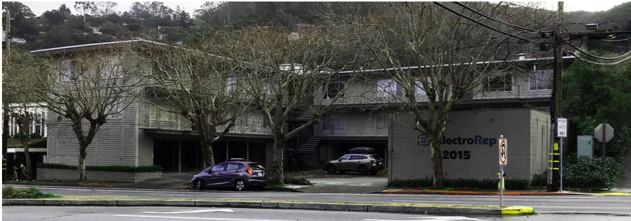
Figure 85. Apartment building at 2015 Bridgeway. Source: David Neuman
