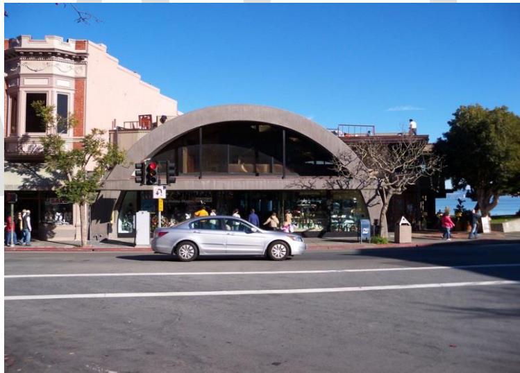
Figure 72. Purity Shops, 660 Bridgeway. Source: Christopher VerPlanck
