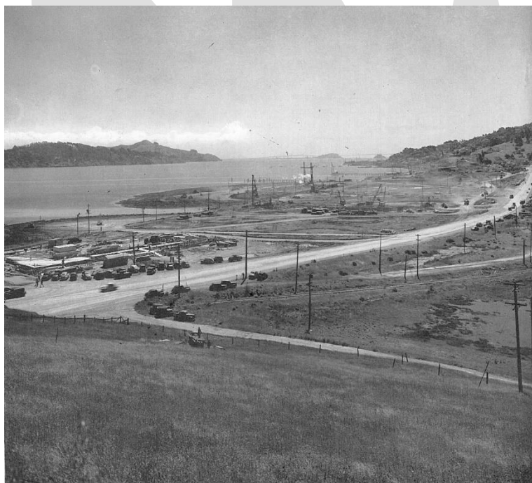
Figure 67. Marinship site being filled and graded, spring 1942. Source: Richard Finnie, Marinship: The History of a Wartime Shipyard
