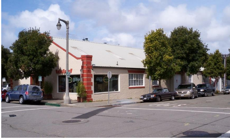
Figure 68. Former Marinship Hiring Hall. Source: Christopher VerPlanck
