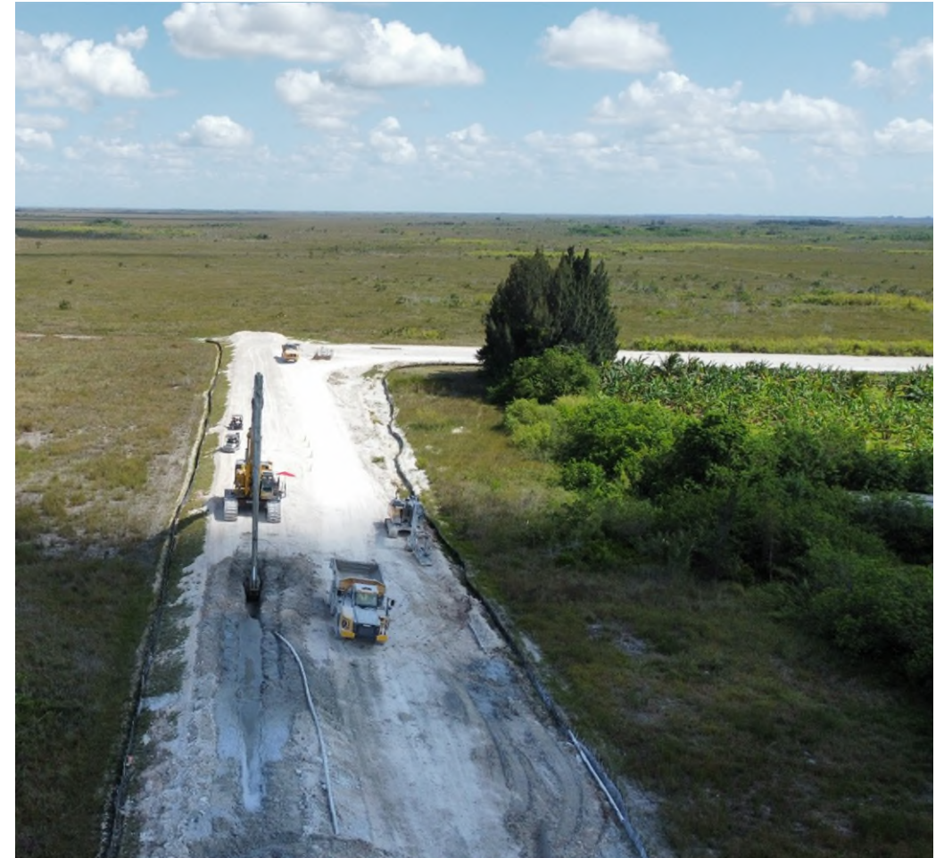
CB Wall Construction
