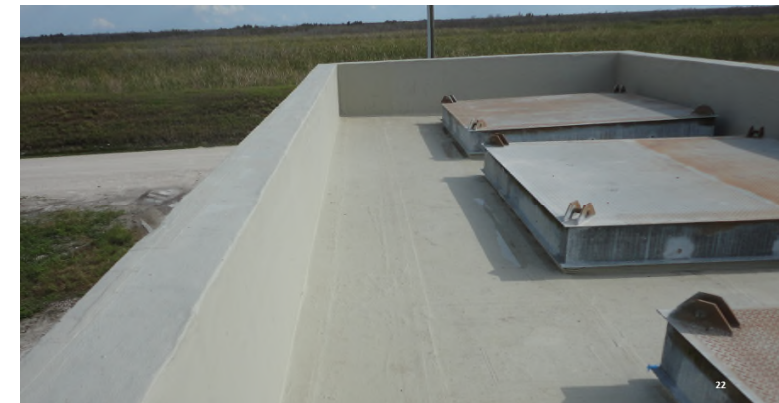
S-250S: Complete roof replaced 652 sq-ft, $104,000
