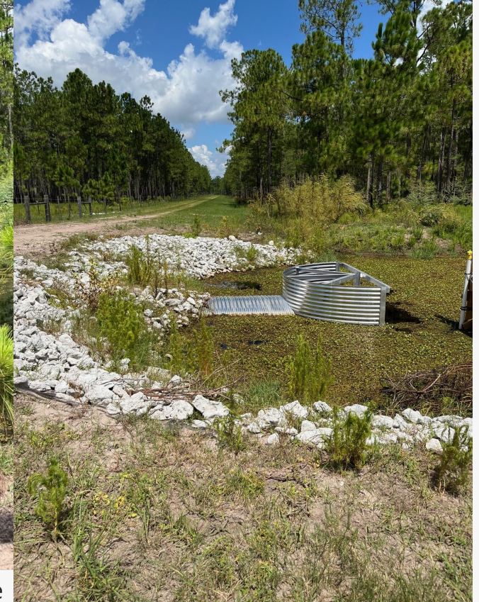
Image of 60" riser culvert replacement in the Big Bend Swamp
