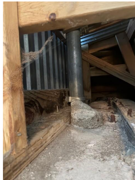
Mast under Tin
