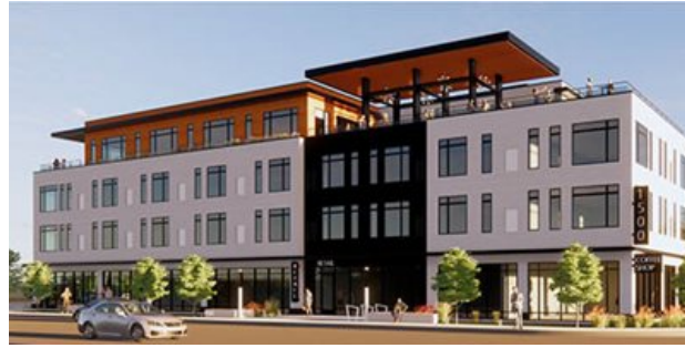
The New Generations development in Brooklyn Center will include affordable housing for veterans and people experiencing homelessness, and will offer support services and youth programming. (Artist rendering.)
