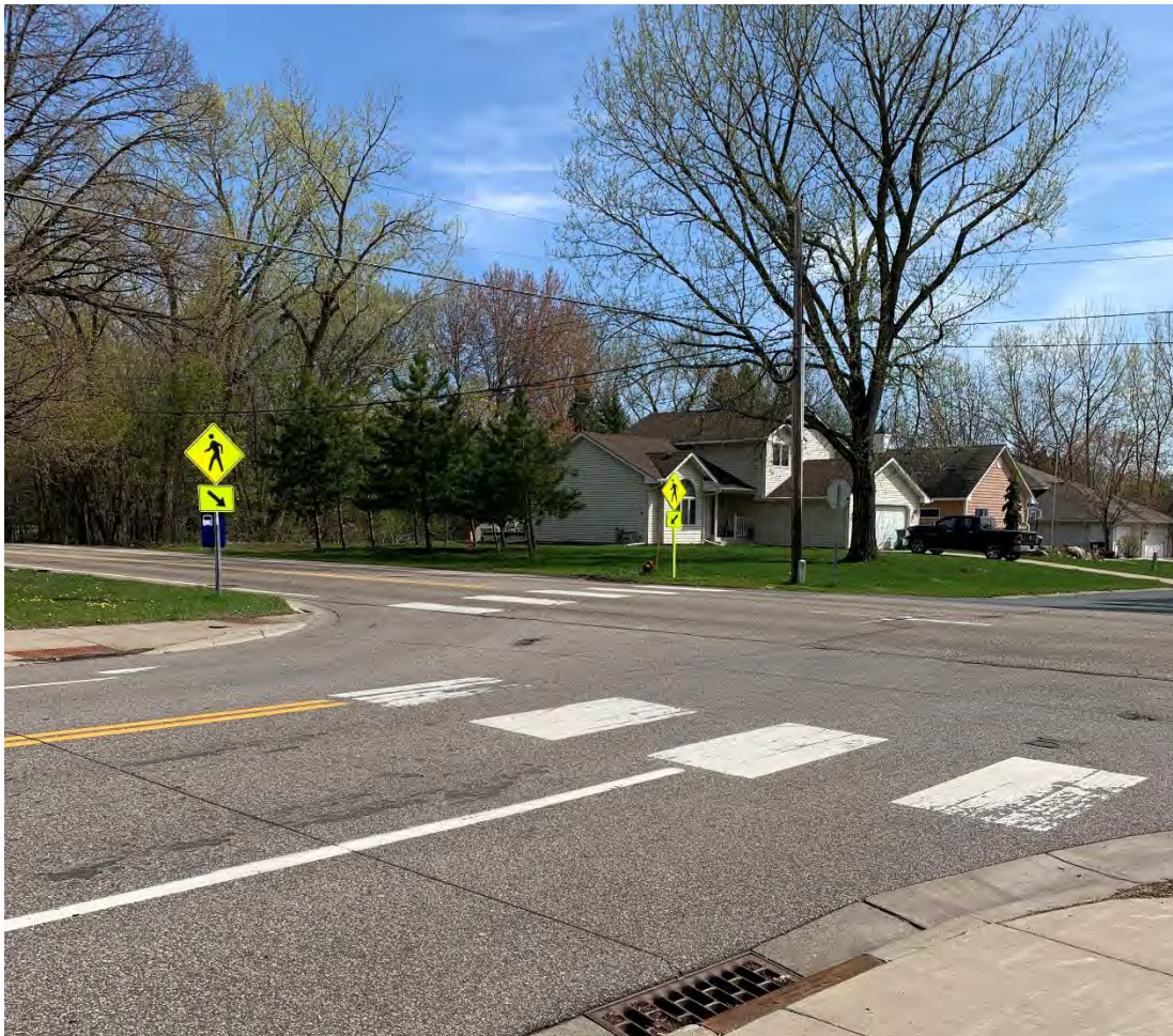
An uncontrolled pedestrian crossing over Victoria Street at W County Rd D.
