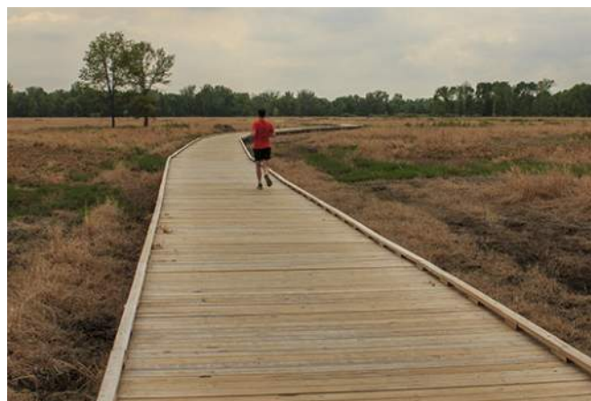
Wetland boardwalk (photo of Blaine Wetland Sanctuary by minnesotaseasons.com)
