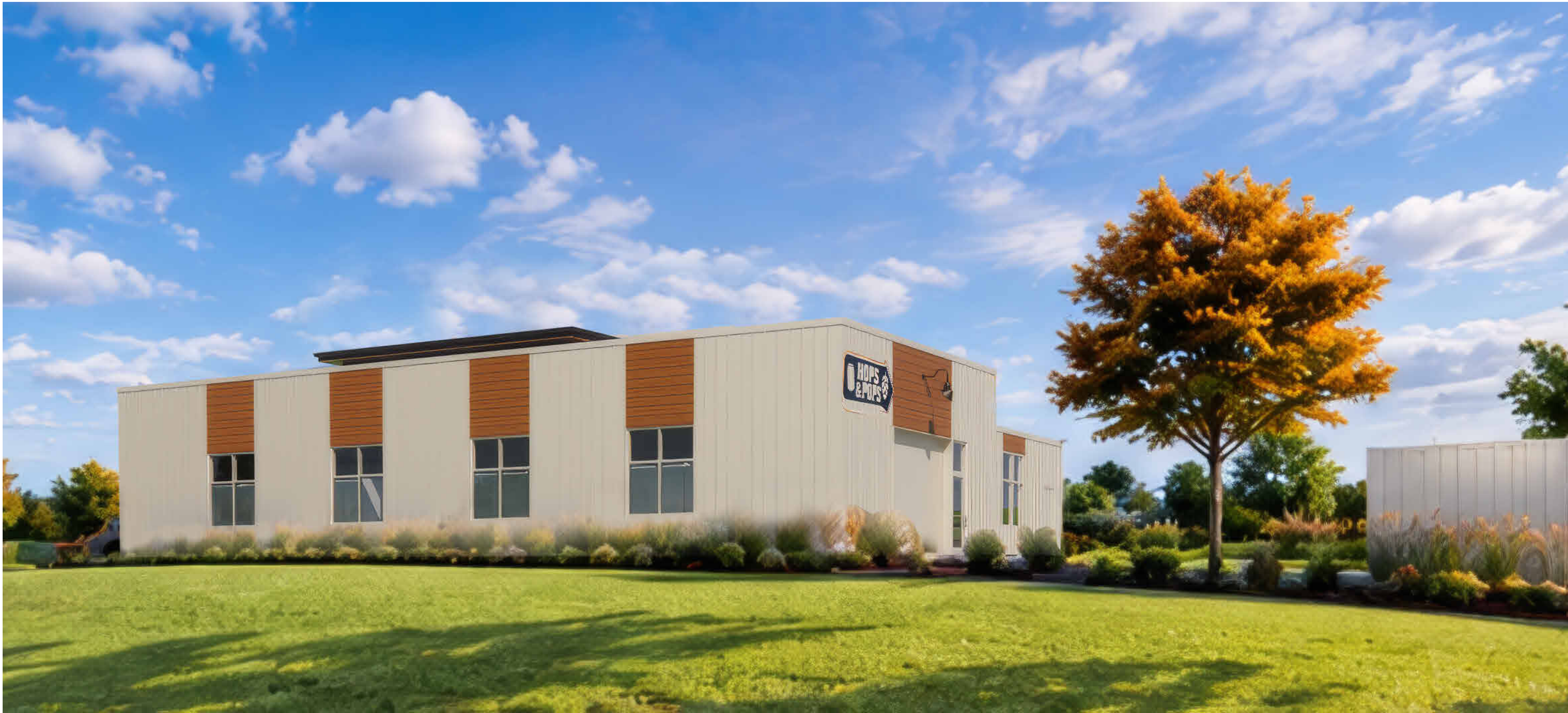
VIEW OF DRIVE-THRU EXIT FROM HWY 60
