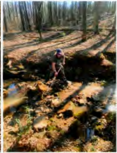
clean-up in progress
