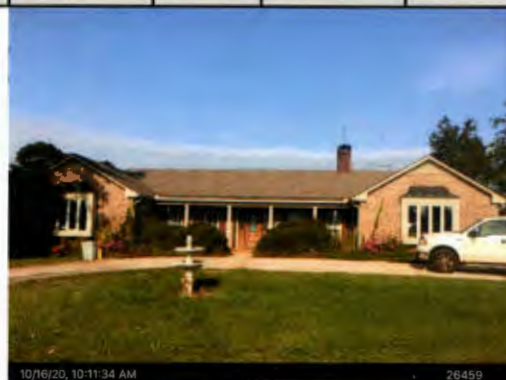
2021 house completely remodeled on the inside after fire per owner.. ab
