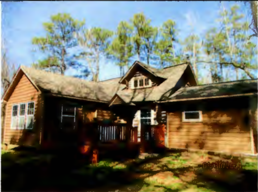
2014: Field Inspection on 9-4-14 after CC issued on 5-27-2014. Changed: to central HVAC; Architectural shingles added bath and extra fixtures, and removed screened porch and added additional heated square footage. HB 9-23-2014.
