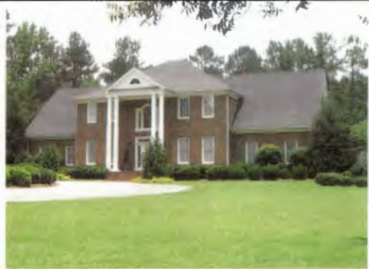
2012: 280sf Fin Attic (right side of house) + 400sf Unfin Attic (left side of house = 680 sf@41% finished - dwg
