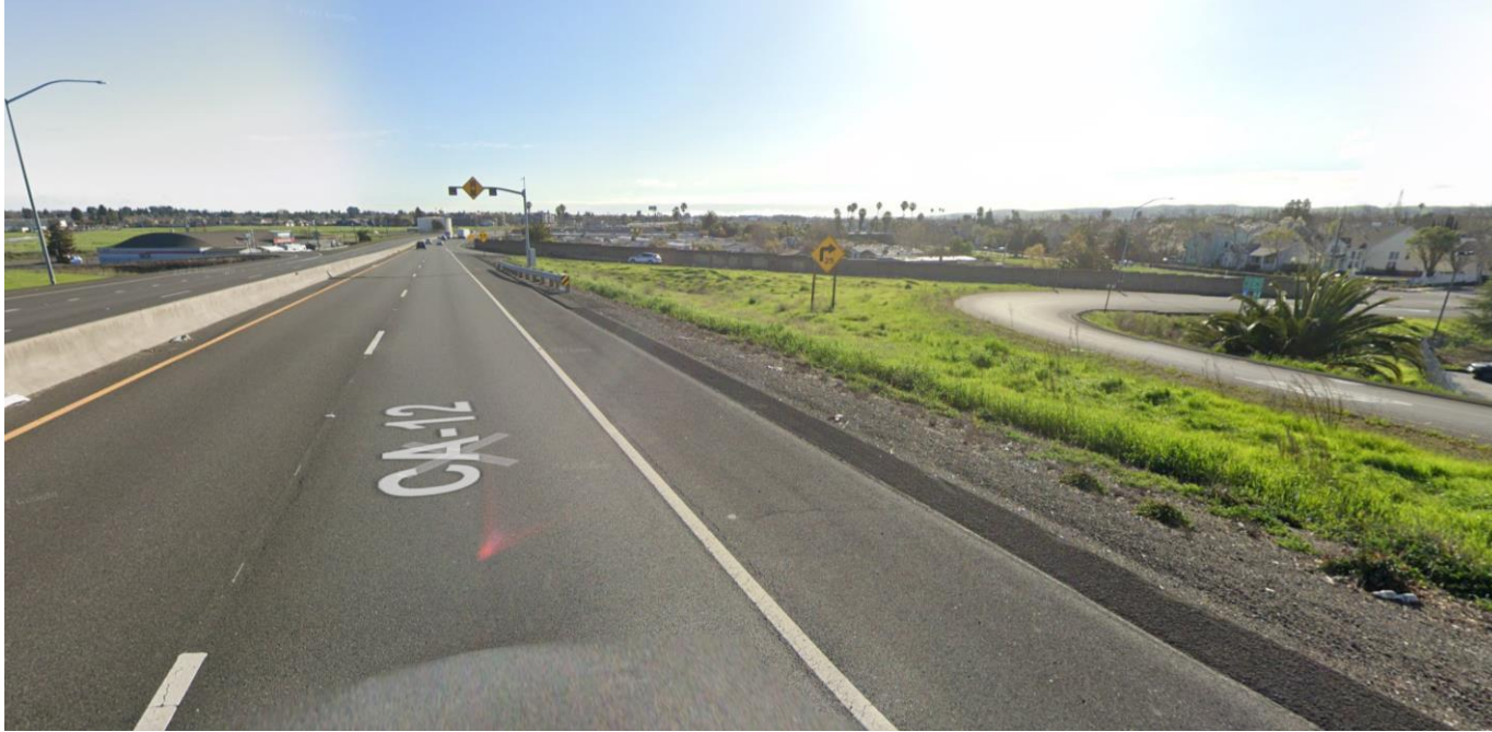
Pre-Construction Photo of the Triangular Area at the Civic Center Boulevard Off Ramp and On Ramp:
