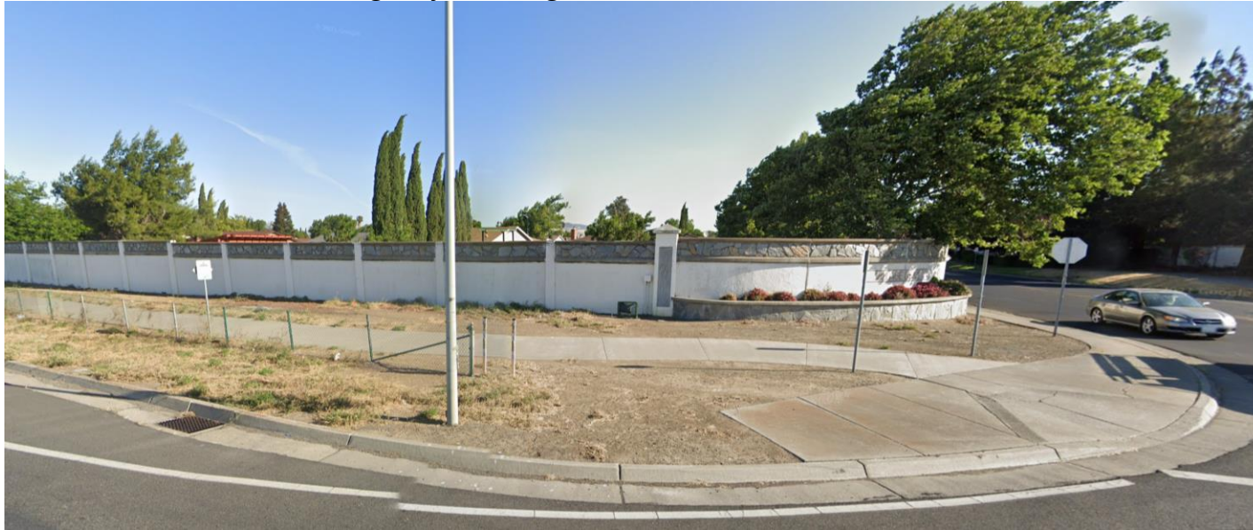
Pre-Construction Photo of the Areas West of the Highway 12/Village Drive Intersection:
