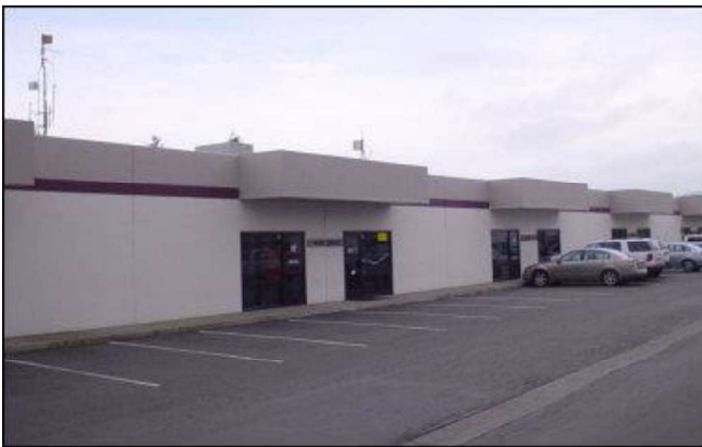
Day Wireless Certified Service Center in Benicia: Complete with service bays, technician workstations, and customer meeting room.
