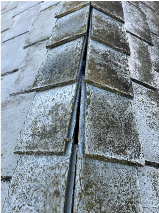
Open Roof Ridge
