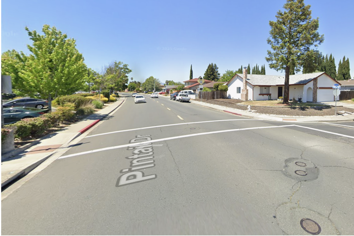
Pre-Construction (Pintail Avenue at Cackling Drive)
