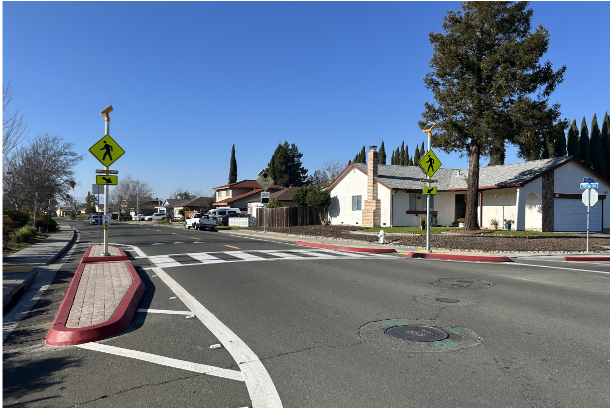
Post-Construction (Pintail Avenue at Cackling Drive)
