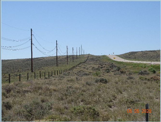
View to the South
