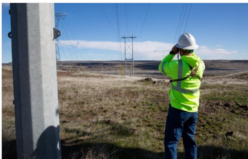
Figure 4-1: Visual Assurance Inspection of Transmission Line
