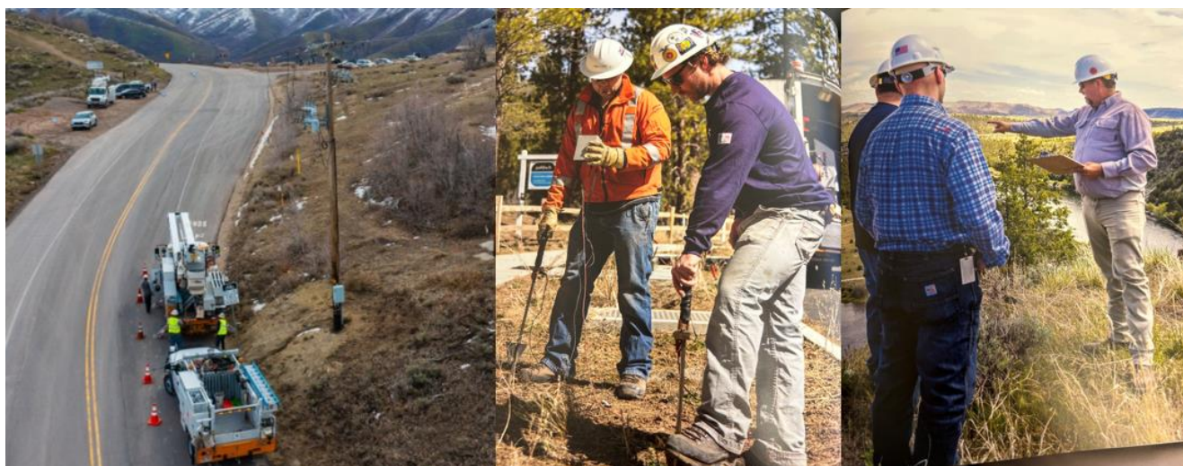
Figure 9-1: Line Workers Performing Work
