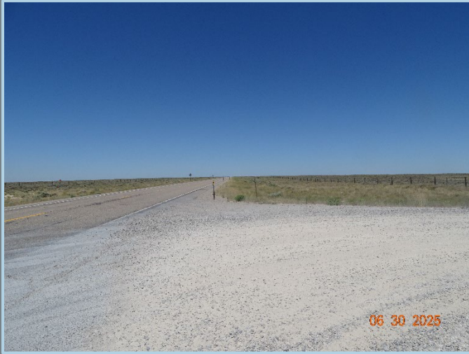
View to the North
