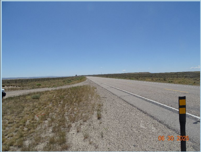
View to the South
