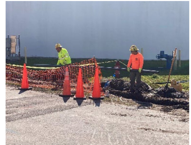
New chemical pipe being installed
