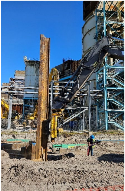
Steel sheeting being installed for deep pump can excavation
