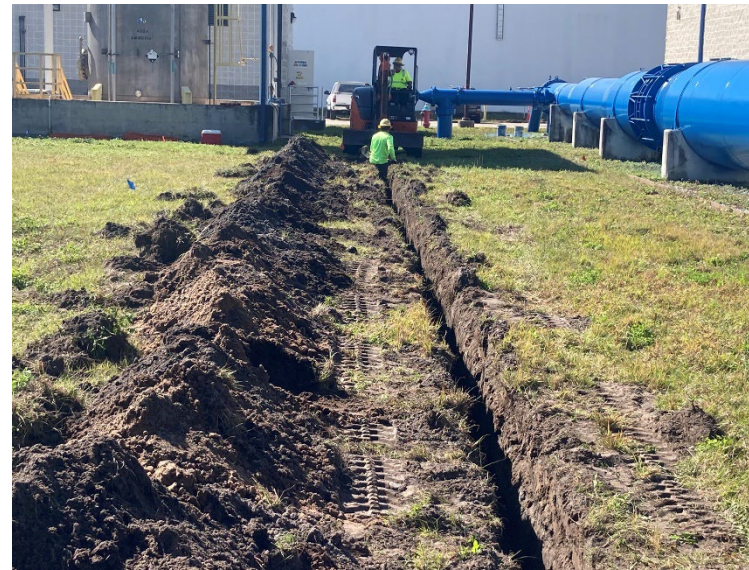
Trench excavation for a new chemical pipe run
