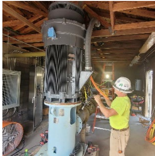
Connecting electric cables to pump motor
