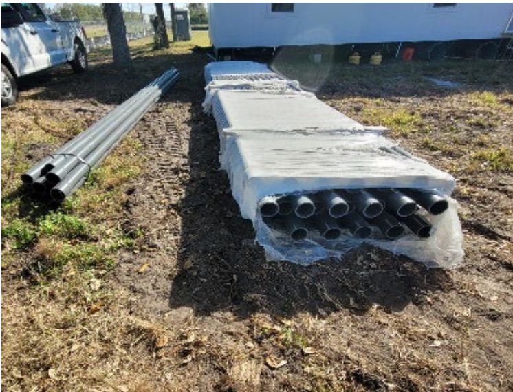
Chemical containment pipe
