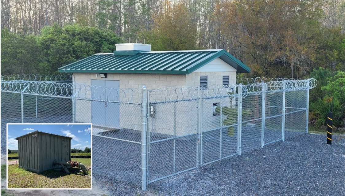
New masonry wellhouse
