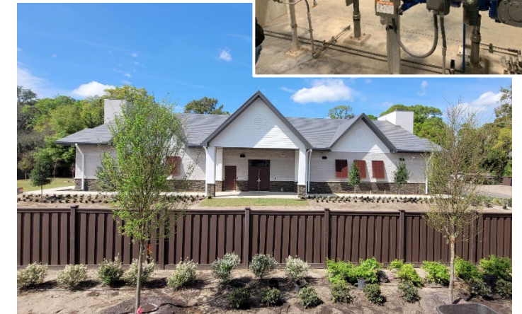
Brandon Booster Station
