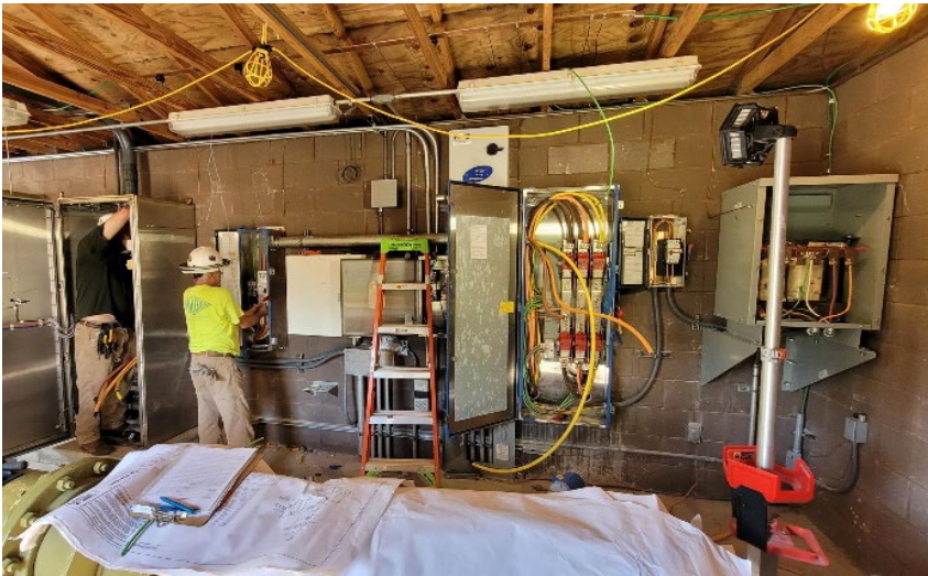
New electrical equipment installation
