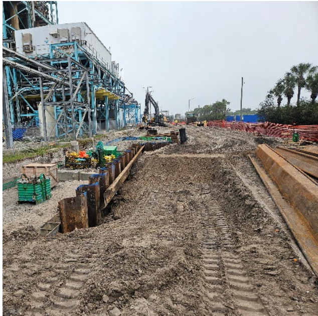
Steel sheeting being installed for deep pump can excavation
