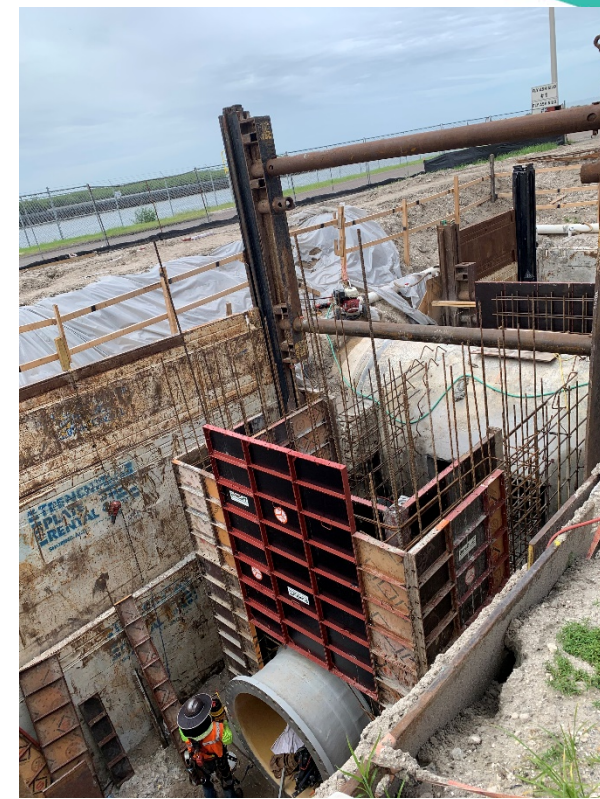
Manhole for valve and 54" stub-out pipe
