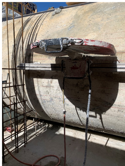
Cut 6' x 6' opening inside of tunnel
