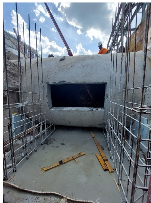
Cut 6' x 6' opening inside of tunnel
