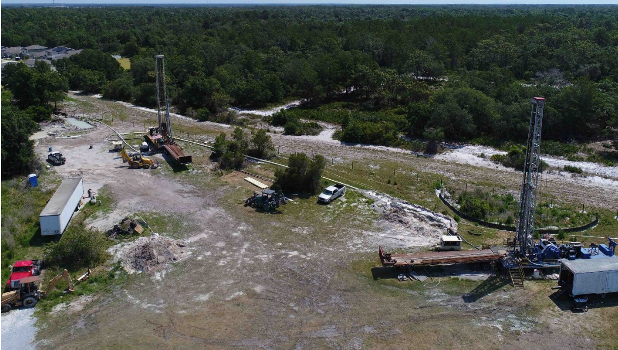
Drill rigs set up for the test well and a monitor well
