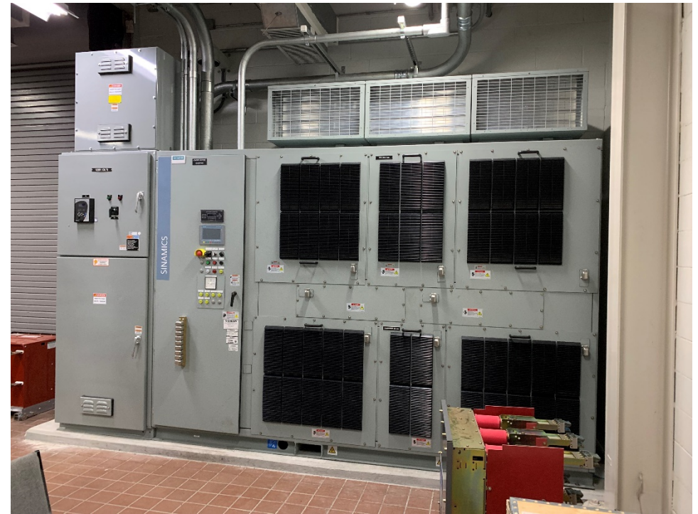
Variable Frequency Drive and Breaker
