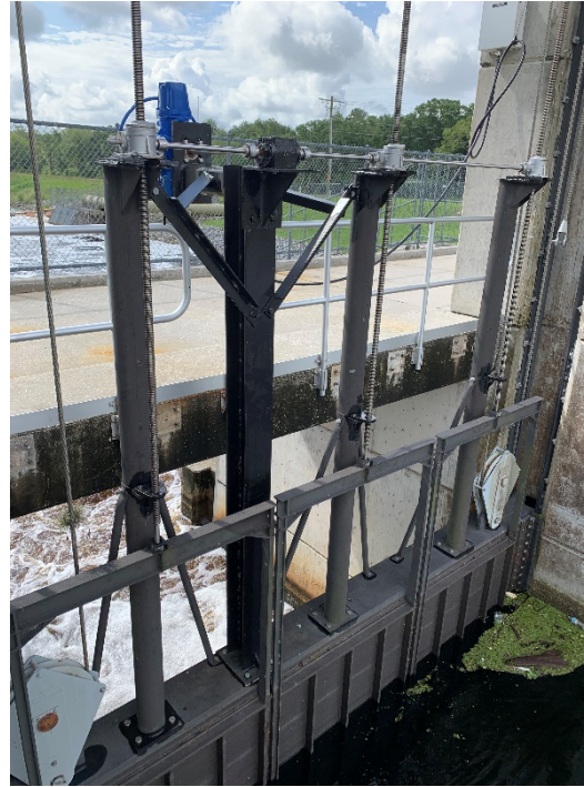
Motorized actuator connected to the gate
