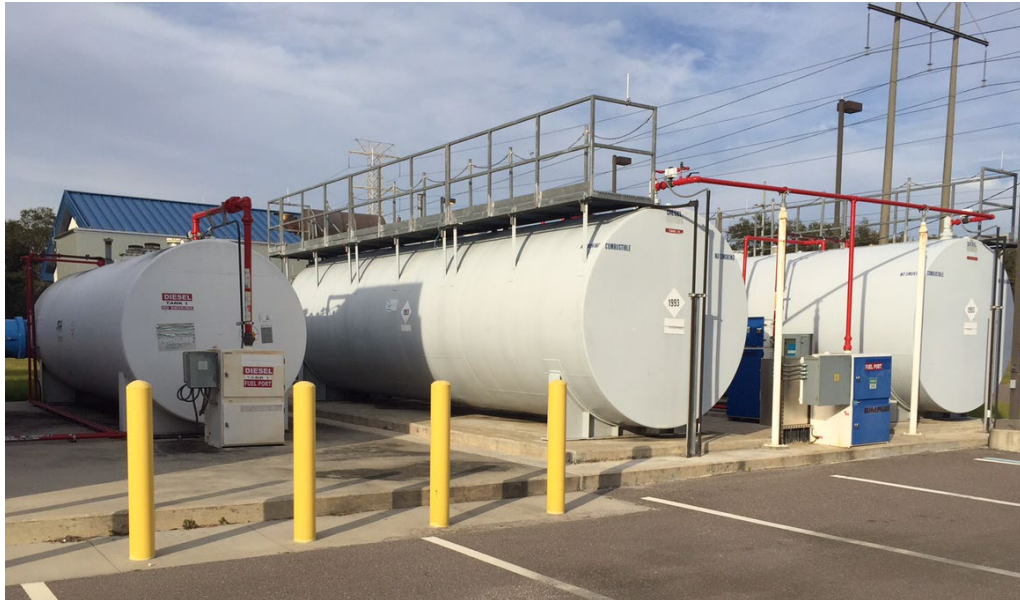
High Service Pump Station diesel fuel tanks
