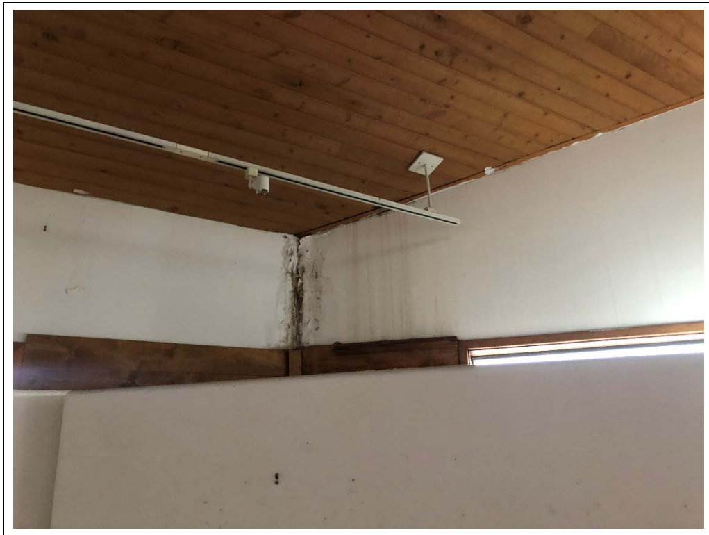
18. Water damage observed on wall/ceiling. (13200-25)
