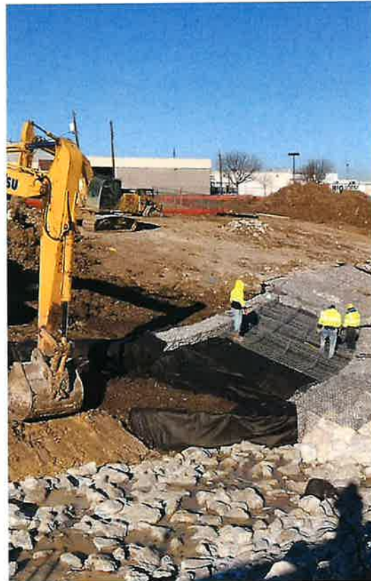
Construction of new north-south drainage channel connecting to Sutton Creek
