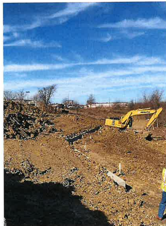
Backfilling completed soldier wall
