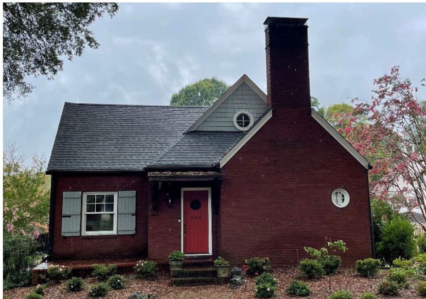
Figure 1. Thompson-Anderson House front elevation
