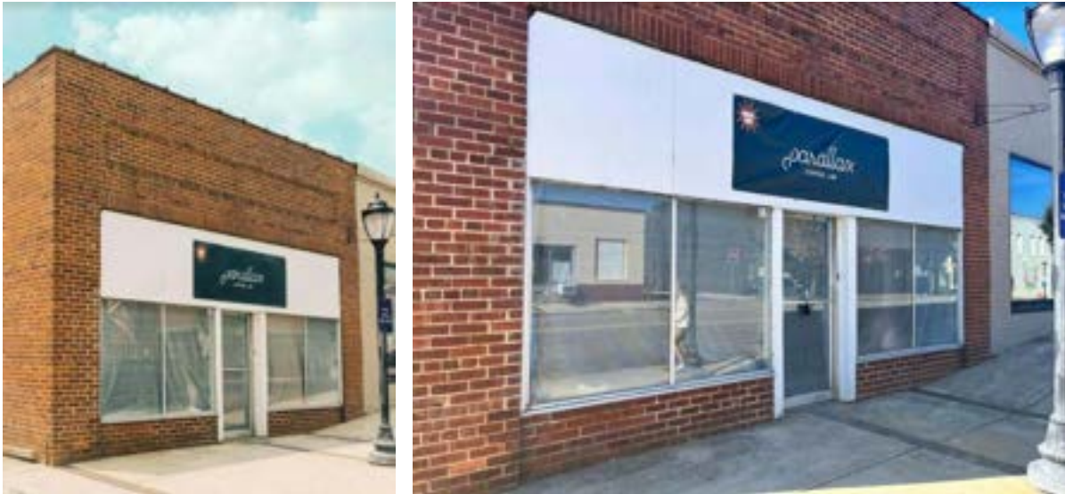
North Façade photos
