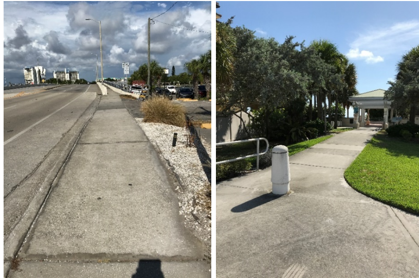
Figure 16: Sidewalk along Eastbound Approach of SR 699 (Left) and Sidewalk towards Beach (Right)
