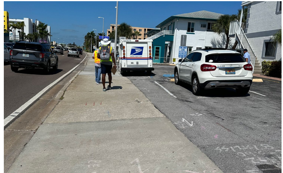
North Segment: Wide and frequent driveway openings were observed in this segment.
