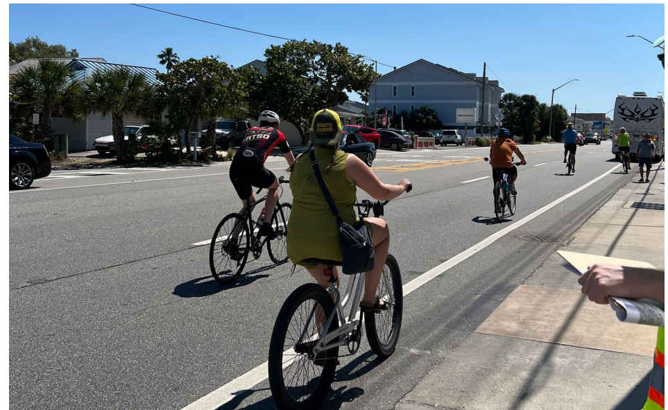
South Segment: Sidewalks are flush with the bike lanes and roadway. Vehicles parked/idling in the outside travel lanes forces bicyclists into the roadway with multiple conflicts.
