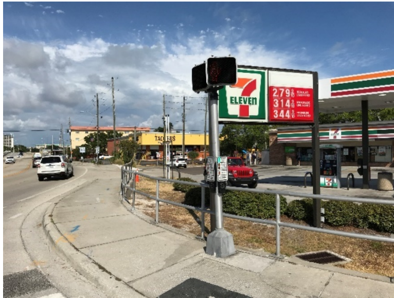
Figure 12: Pedestrian Signal at Intersection of West Gulf Boulevard and SR 699
