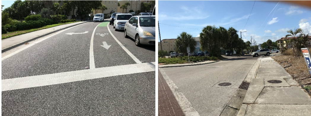
Figure 8: Pavement Markings on Eastern Approach of SR 699 at Intersection of 1 st Street / West Gulf Boulevard (Left) and Southern Approach of 1 st Street (Right)
