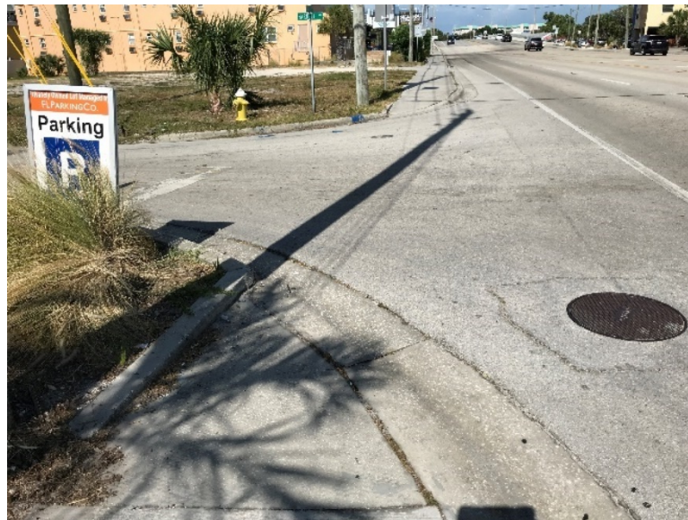
Figure 13: Curb Ramps at Southern Approach of Harrell Avenue
