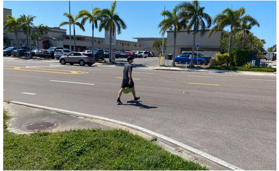
Central Segment: Frequent crossings at unmarked crosswalks were observed at 108th Avenue.
