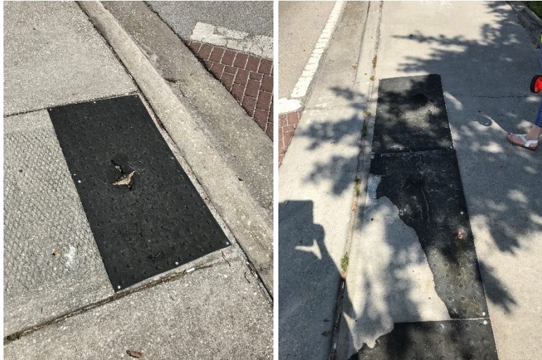
Figure 14: Detectable Warning Mats at Intersection of SR 699 and 1 st Street / West Gulf Boulevard
