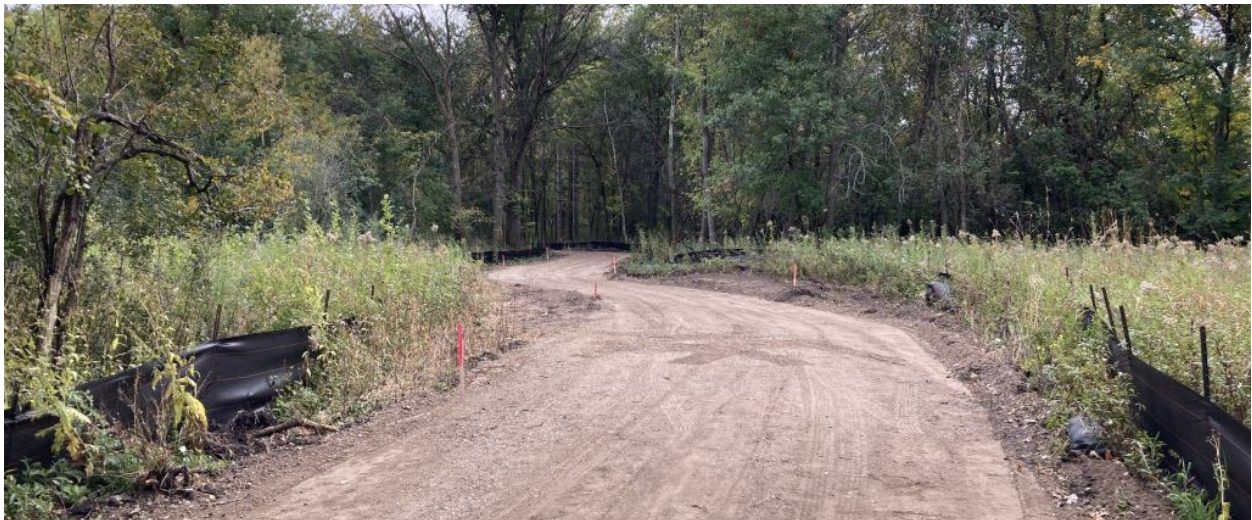
Rush Creek Regional Trail – Construction of reroute underway and ready for pavement.
