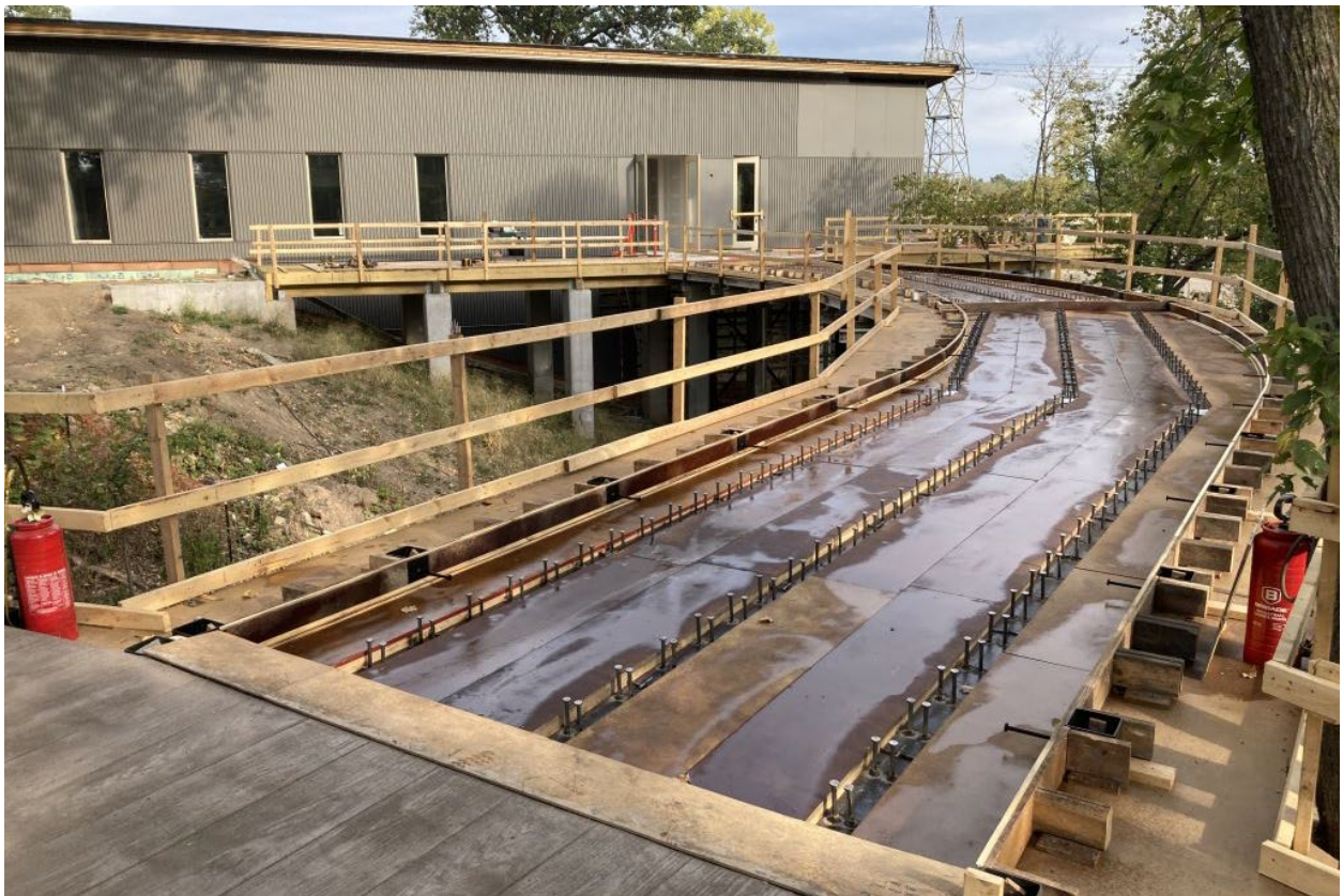
Treetop Trail – Preparing for final concrete pour at connection to Gateway Center.
