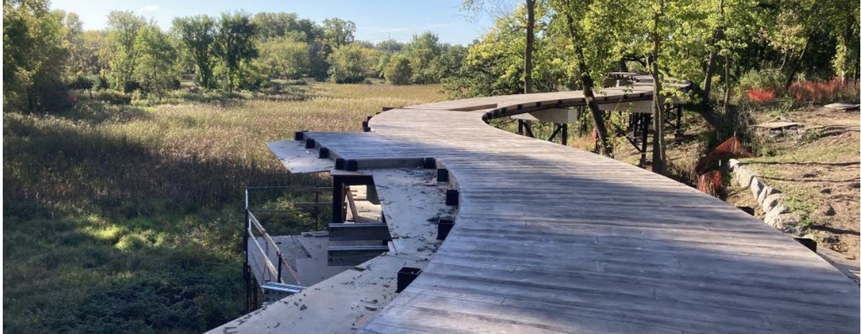
Treetop Trail – Completed segments continue.
