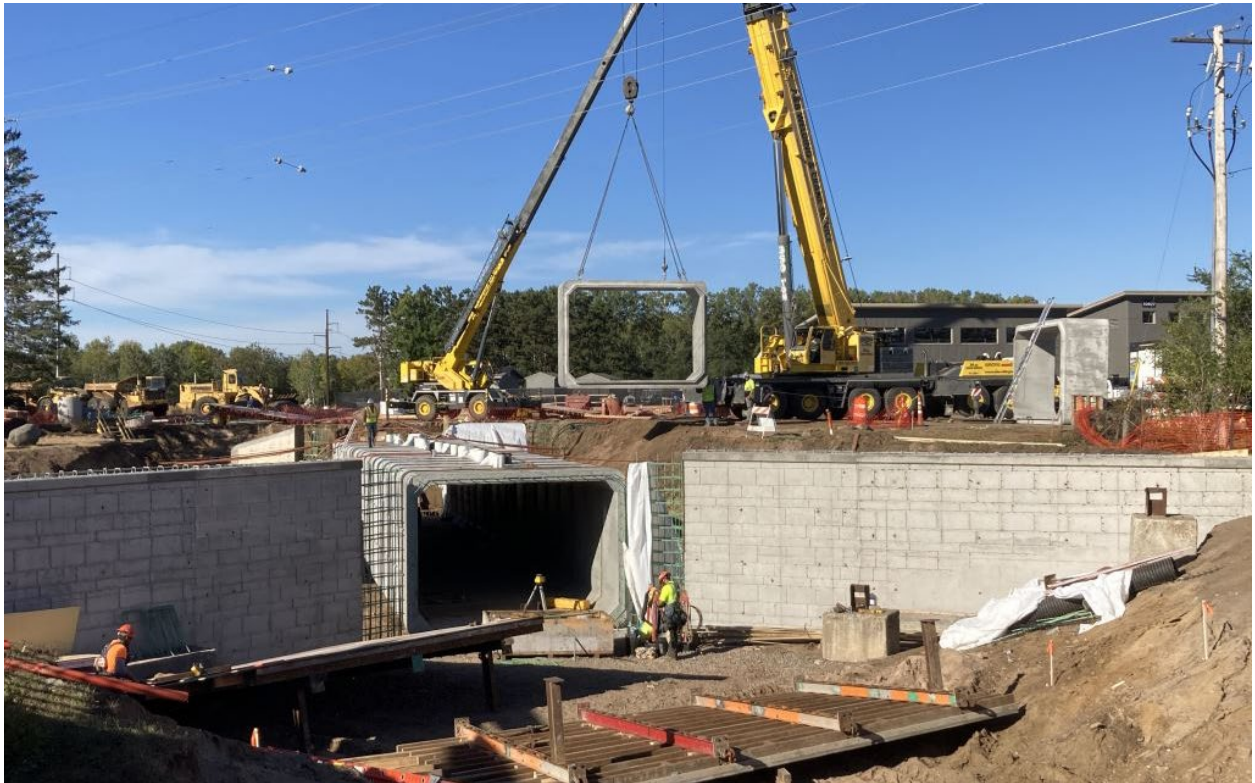
Underpass – Placement of culvert boxes in process.
