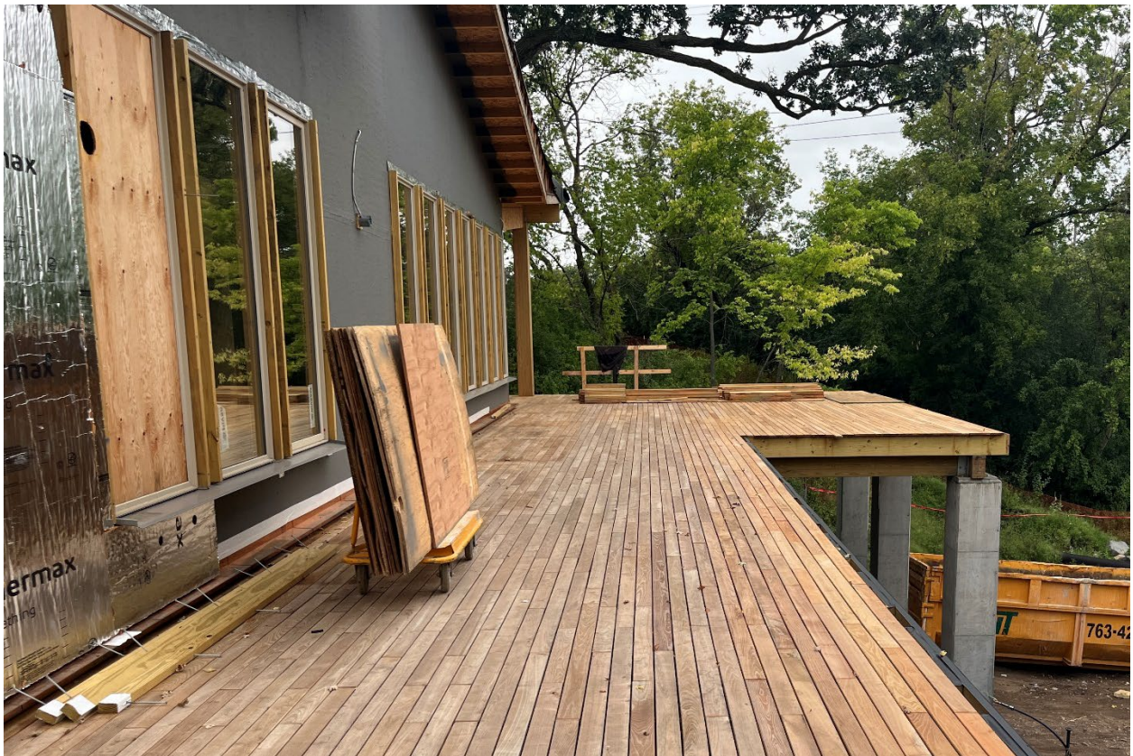
Gateway Center – Riverside decking in place.
