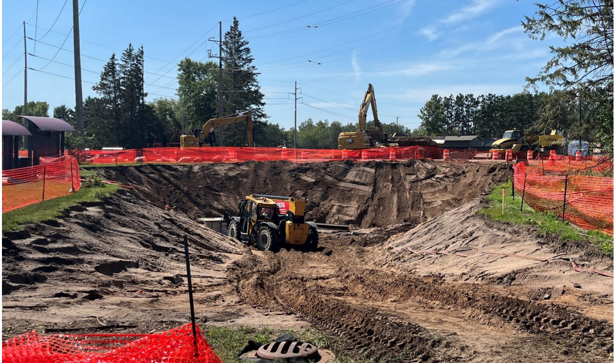
Underpass – Excavation for tunnel in process.
