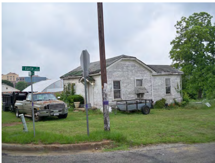
VIEW OF THE DWELLING ON THE PROPERTY
