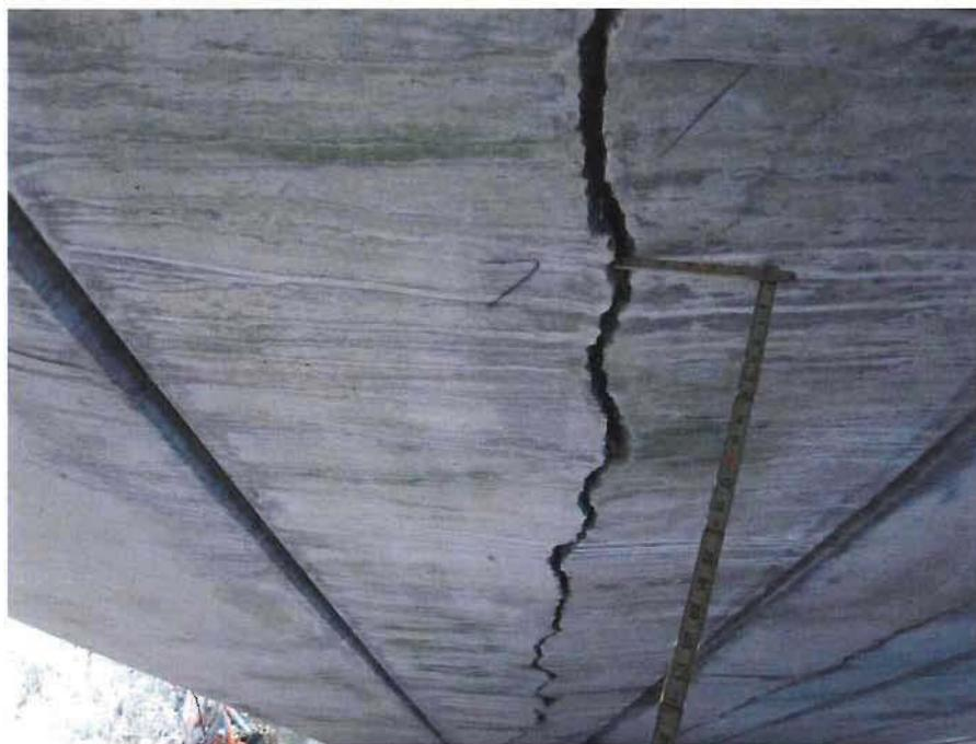
13. Beam 7, note the crack width up to 1".
