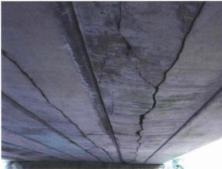
12. Beams 6 and 7, looking ahead. Note the wide longitudinal cracks.
