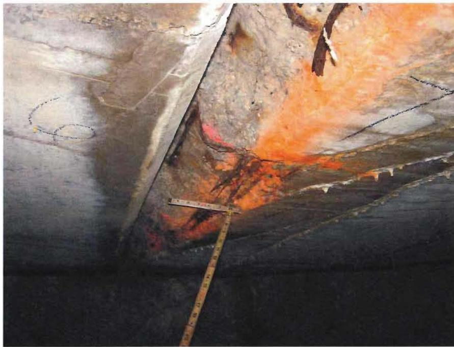
14. Beams 6 and 7 at the far abutment, looking ahead. Note the wide longitudinal cracks, radiating cracks and the spall with exposed severely rusted prestressing strands.
