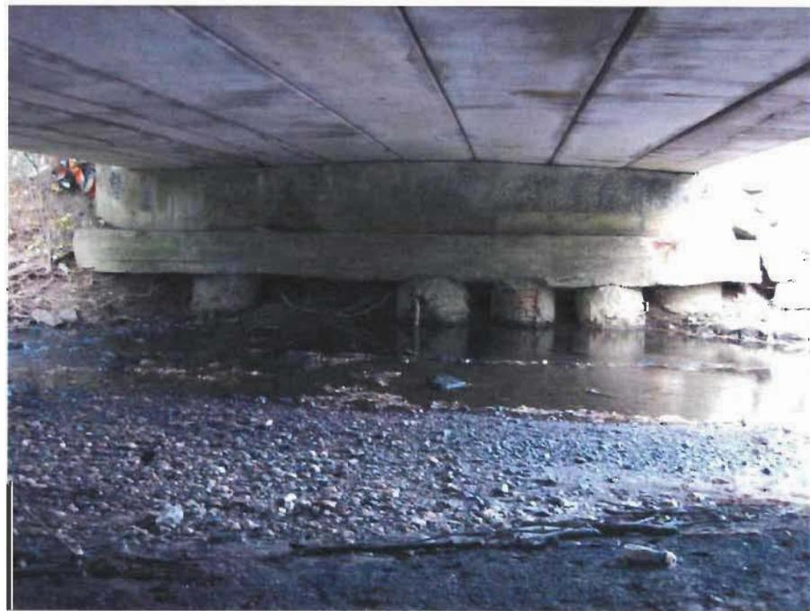
16. General view of the near abutment, looking back. Note the undermined footing and exposed concrete caissons.
