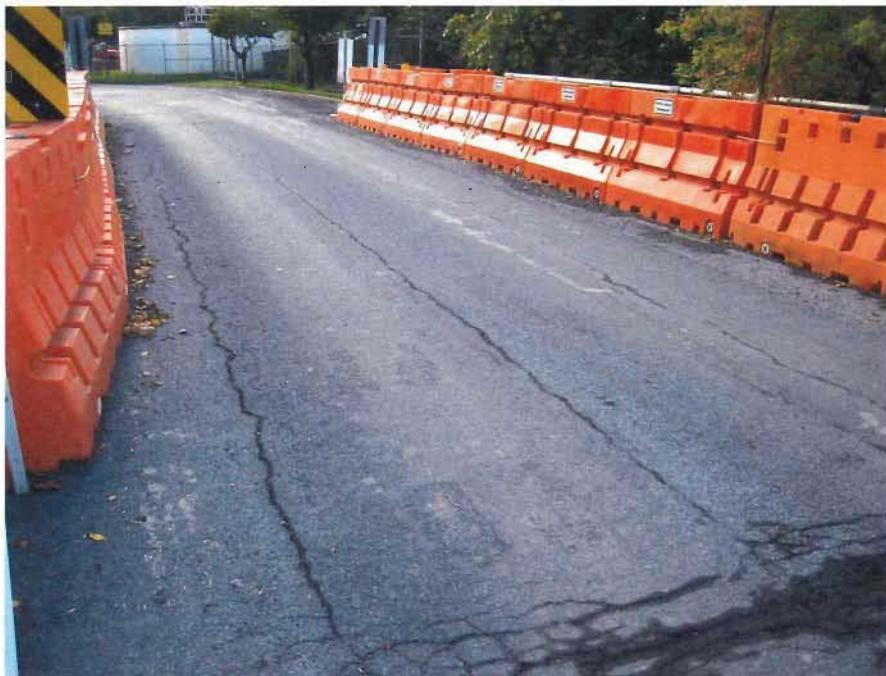
5. General view of the deck wearing surface, looking ahead. Note the reflective cracking.
