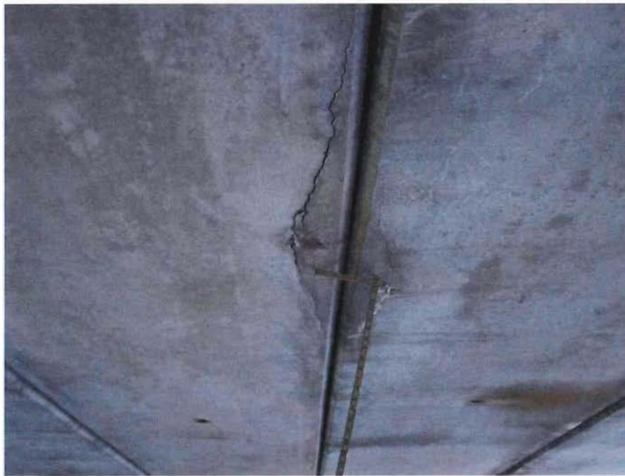
10. Beams 3 and 4, near mid-span, looking back. Note the incipient spalls.
