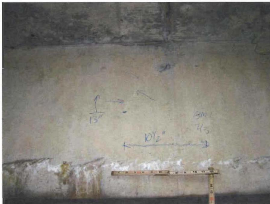
7. Beam 1 beneath the parapet deflection joint at the 2/3 span point. Note the diagonal crack in the beam web.
