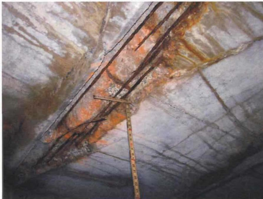
11. Beam 6 at near abutment, looking back. Note the severed and rusted prestressing strands.
