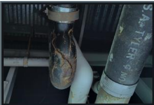
Broken Sanitary Drains in Need of Replacement.
