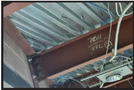
Poor Steel Connection (Knife Joint)
