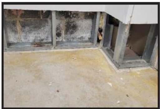
Exterior CMU Block in need of Damp Proofing at below grade locations.
