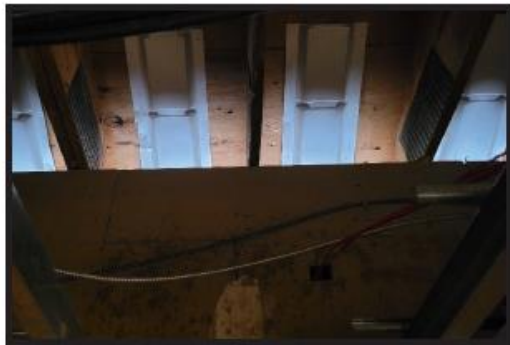
Photo Taken from the Interior Shows Eaves Wide Open to the Outside.
