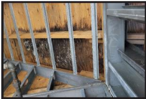
Wood Sheathing at Interior Roof Line in Need of Replacement. Water Infiltration Needs to be Addressed.
