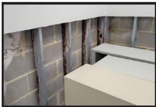
Interior Water Damage from Exterior at Below Grade Locations.
