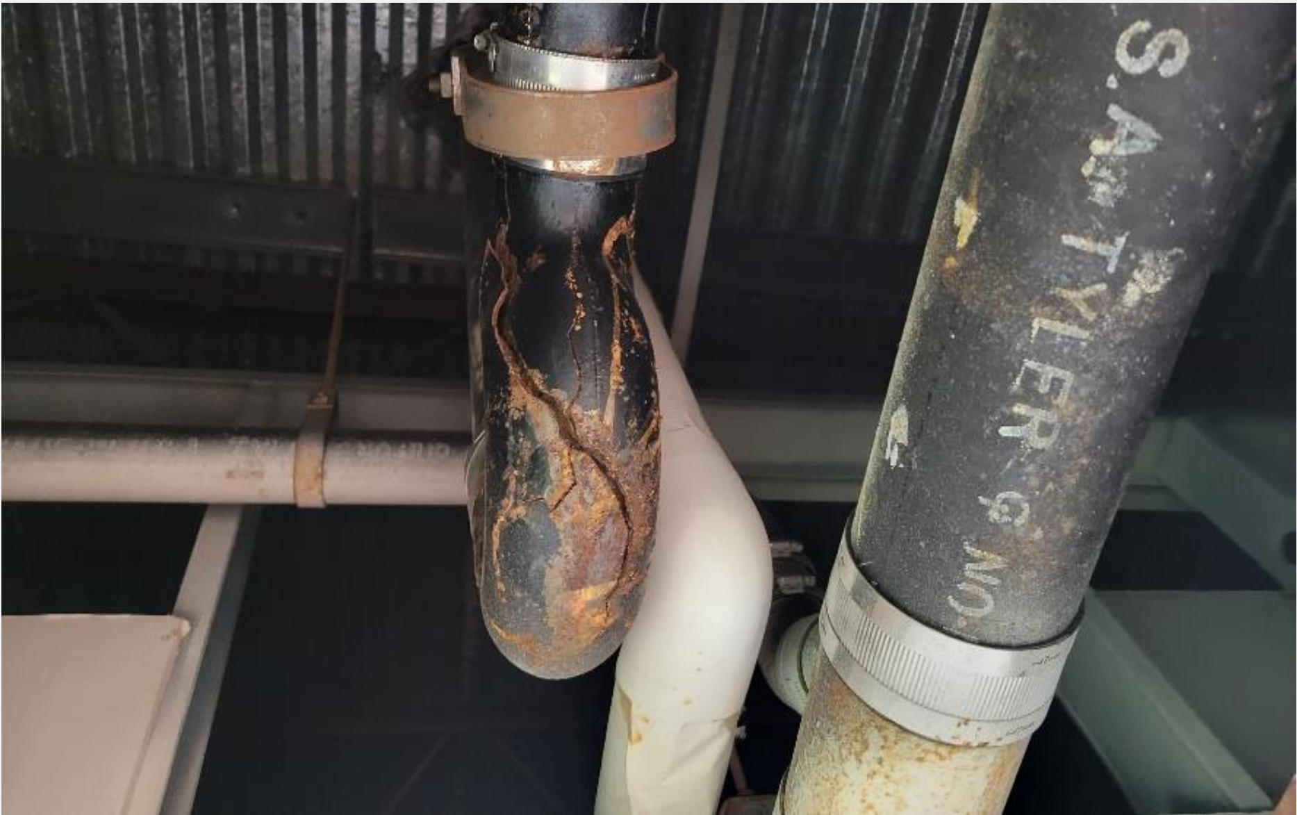
Broken Sanitary Drains in Need of Replacement
