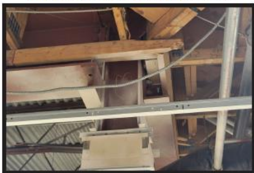
Wood Sheathing at Interior Roof Line in Need of Replacement. Water Infiltration Needs to be Addressed.
