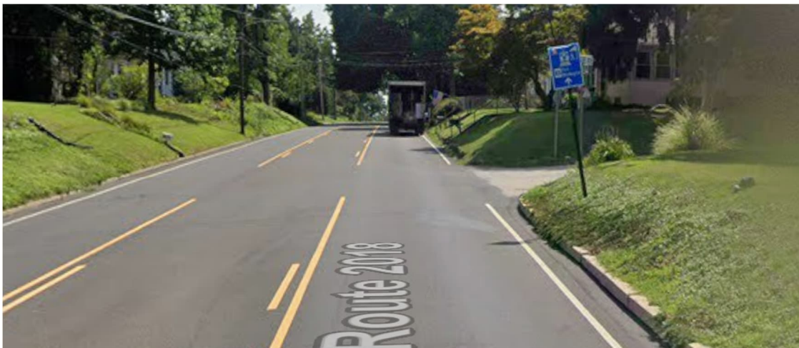
Figure 2: Banks at intersection of Bethlehem Pike and Ellerslie Avenue restrict driver’s view of vehicles parked on Ellerslie Avenue.
