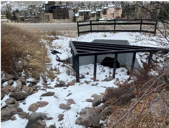
9. Middle Creek culvert that flows under I-70 Frontage Road, looking south.
