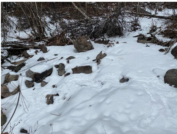
11. Middle Creek upstream of I-70 Frontage Road, looking north.
