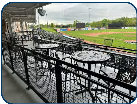
Installation of the Left Field Party Deck completed in FY 24/25
