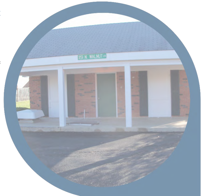
Walnut Lift Station
