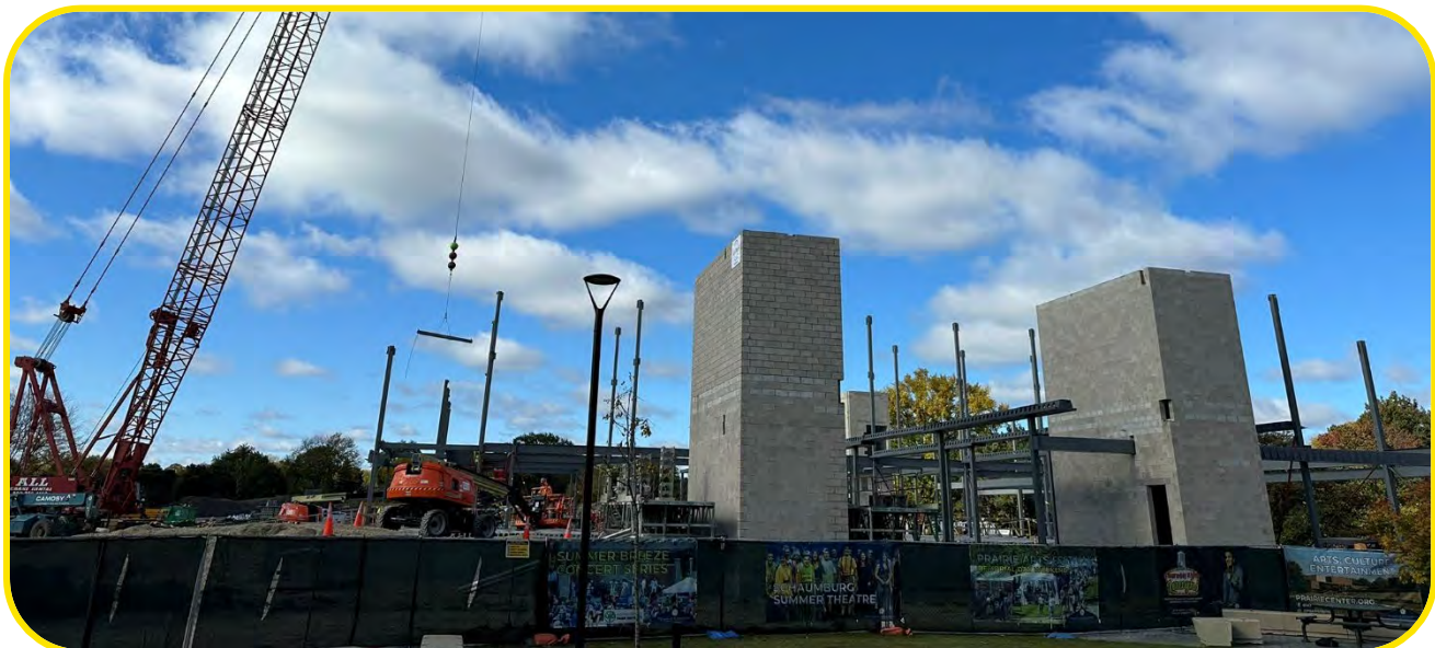
Construction progress of the New Village Hall as of October 2025
