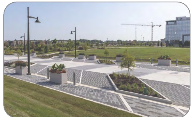
The village's 90 North Shared Street completed in FY 25/26.
