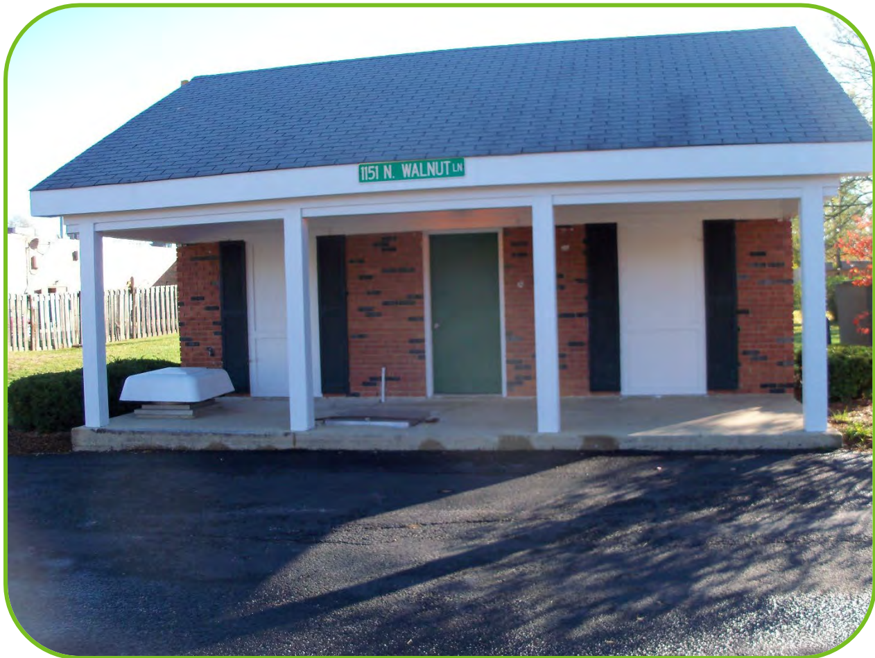
Walnut Lift Station – Scheduled for rehabilitation in FY 26/27
