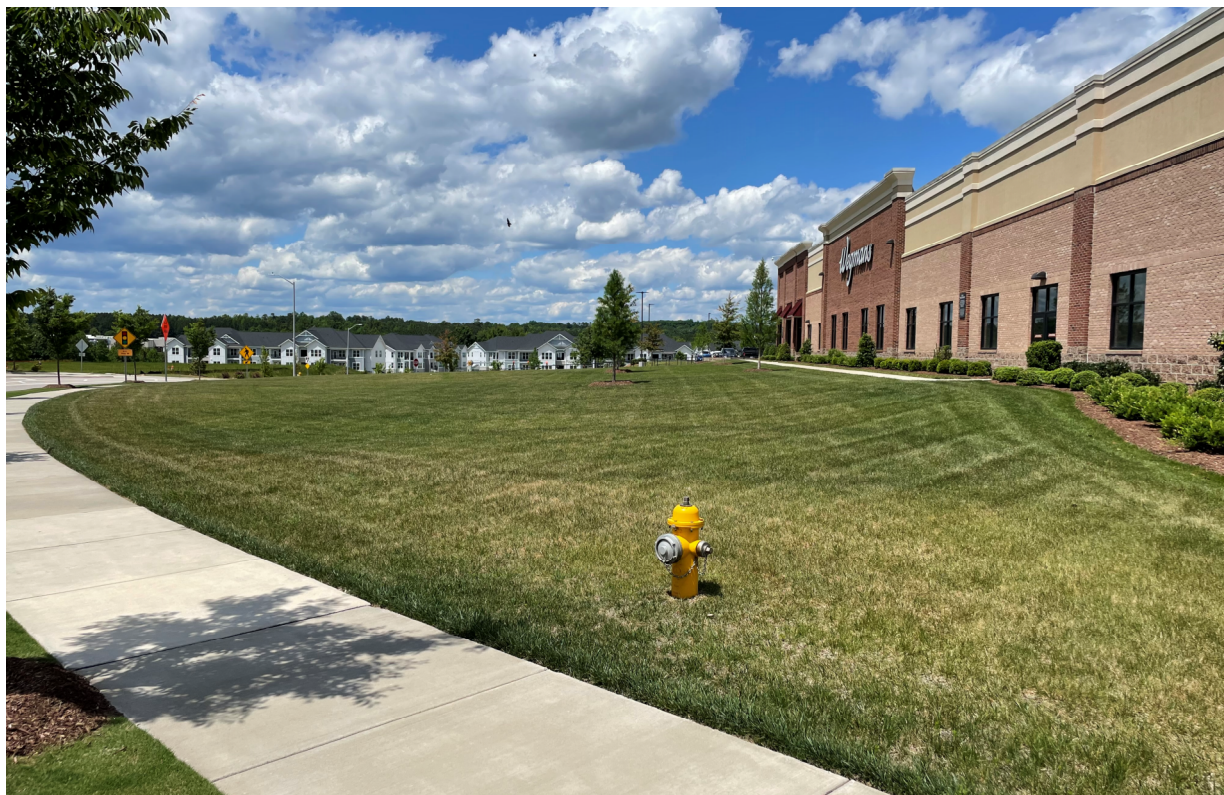
Figure A3 – Existing Condition Photo
