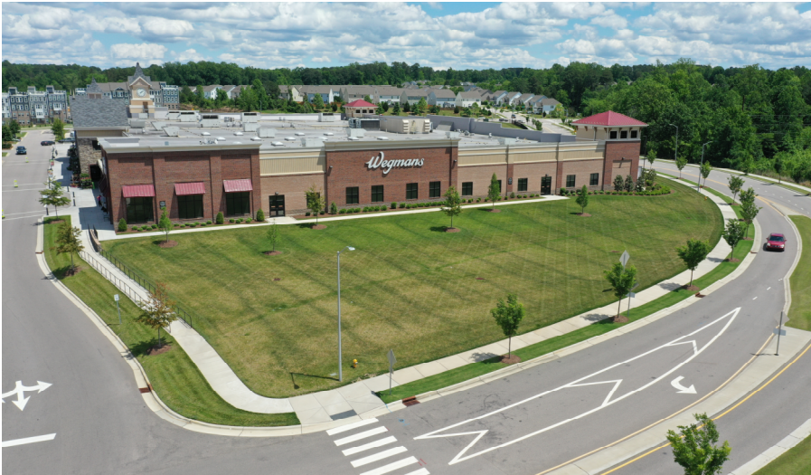
Figure 2 – Existing Condition Photo
