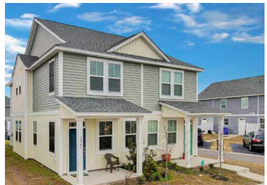
This duplex home in an affordable housing development in North Charleston, SC provides affordable housing.
