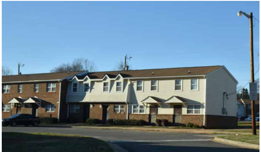
Multi-family public housing complex
