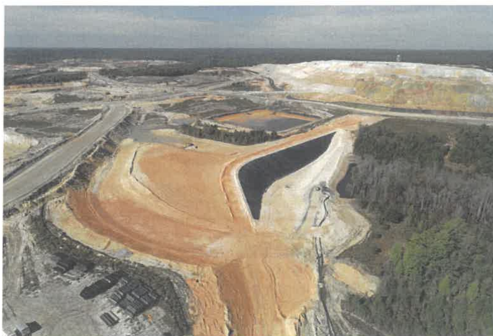
Aerial of HGM Fresh Water Storage Dam
