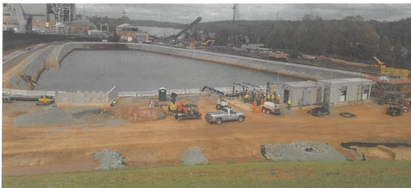
Project operating shortly after completion of construction.
