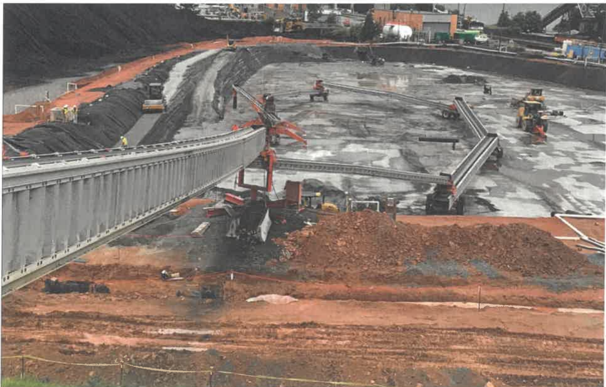
RCC placement at the base and on the side slopes almost complete. Articulated conveying system shown here was used to convey the RCC from the mixing plant to the point of placement for the entire project.
