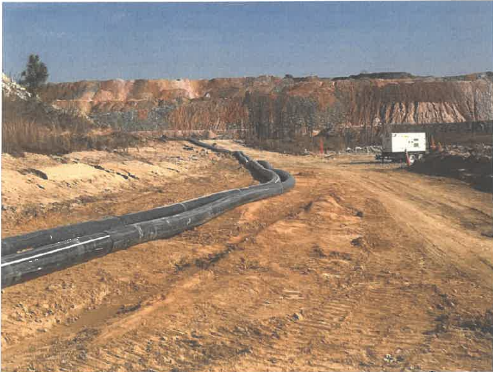
Bypass Pumping of Existing Stream
