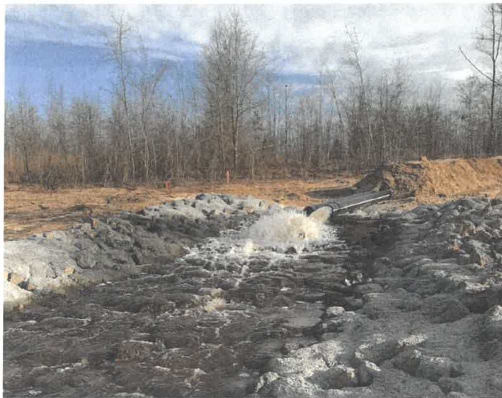
Grouted Riprap Apron at End of Bypass
