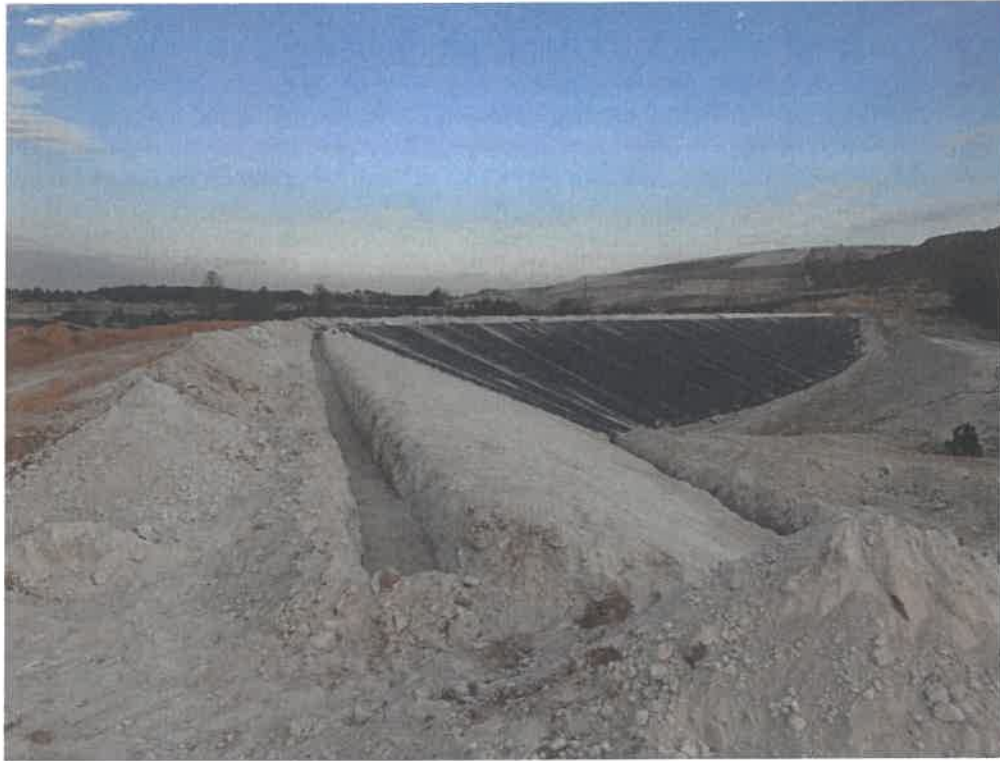
Anchor Trench for Liner Installation
