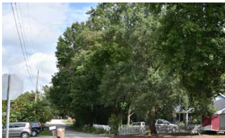
Numerous streets with the study area lack safe/ appropriate pedestrian/ bicycle facilities
