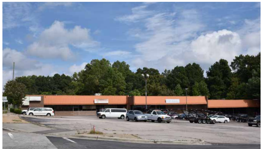
Shopping center along N. White Street just north of the CVS
