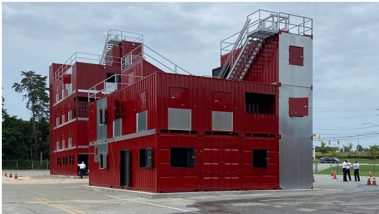
Figure 12: City of Greensboro Fire Training Facility Adjacent to Hospital and Residential:
