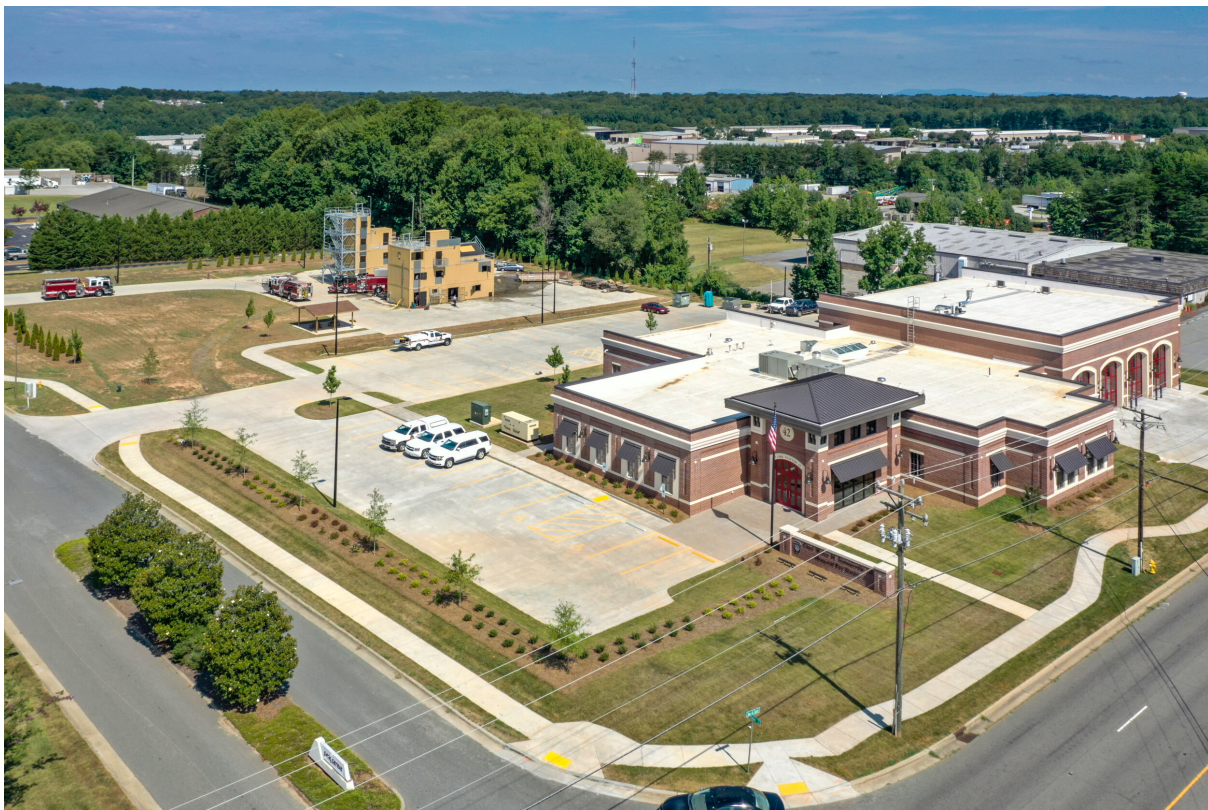
Figure 11: Town of Kernersville, NC Combination Fire Station and Fire Training Facility:
