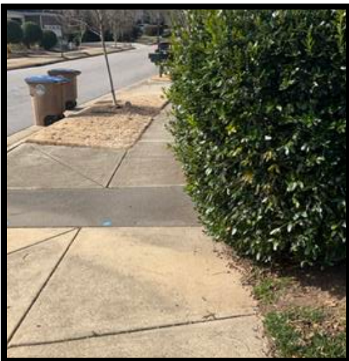
Location: Hertiage Hills Way
