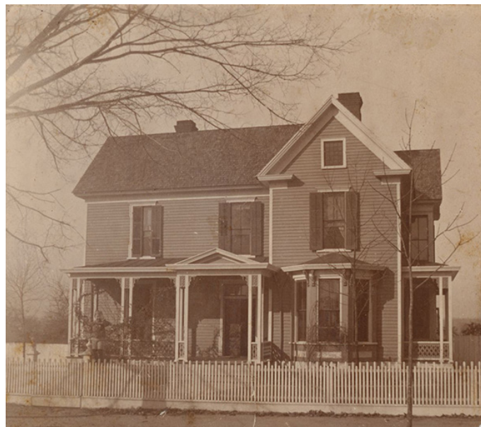
Figure 42. House at 427 North Main Street, which was destroyed by a fire in 2015. Fire is often a challenge experienced in historic preservation.
