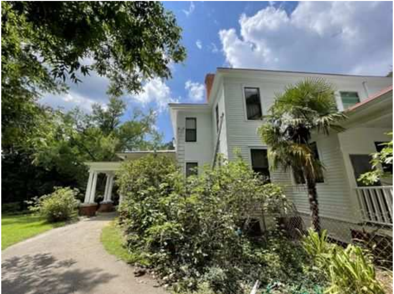
EXTERIOR - Southeast Corner
